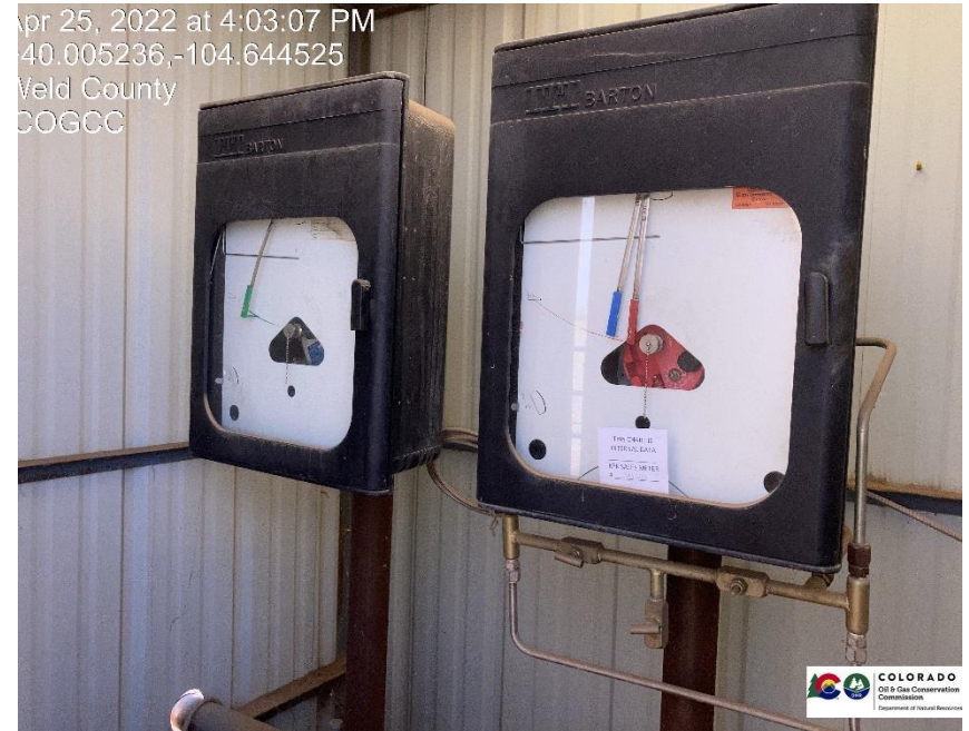
Pic 4 gas meter run is not calibrated
