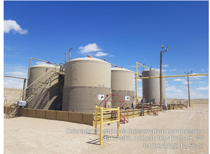
Photo 2 – Produced Water Tank Battery
