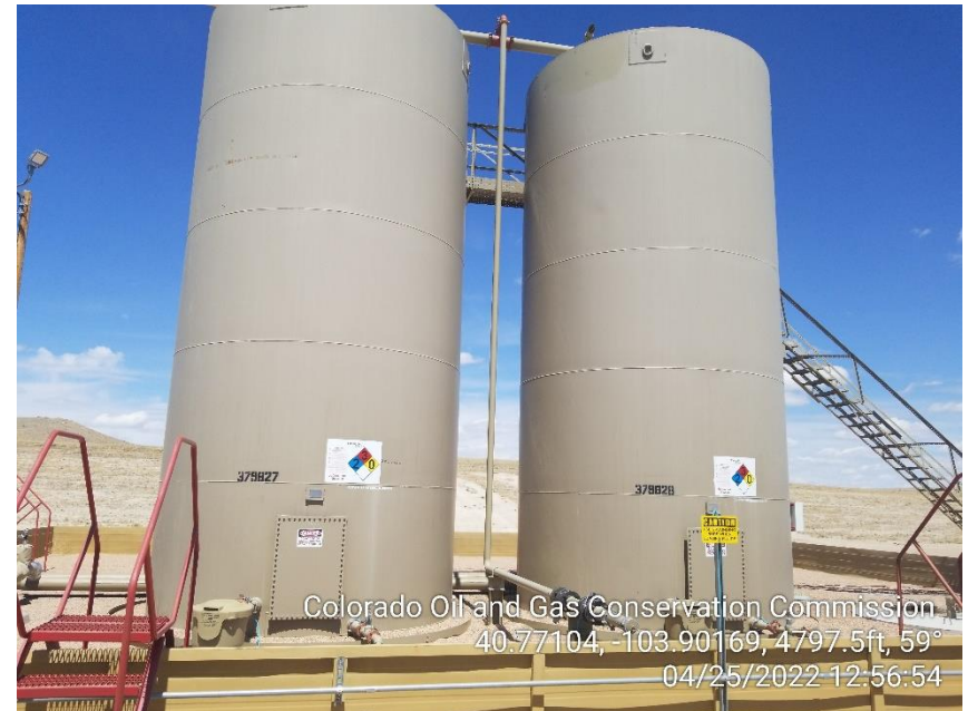
Photo 4 – Crude Oil Tank Battery
