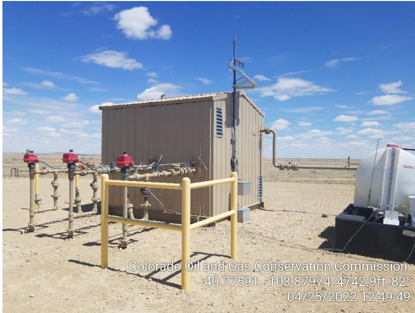
Photo 9 – Gas Lift Injection Meter Shed
