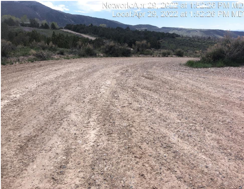
Photo #6586 Insufficient tracking BMP at entrance to location.
