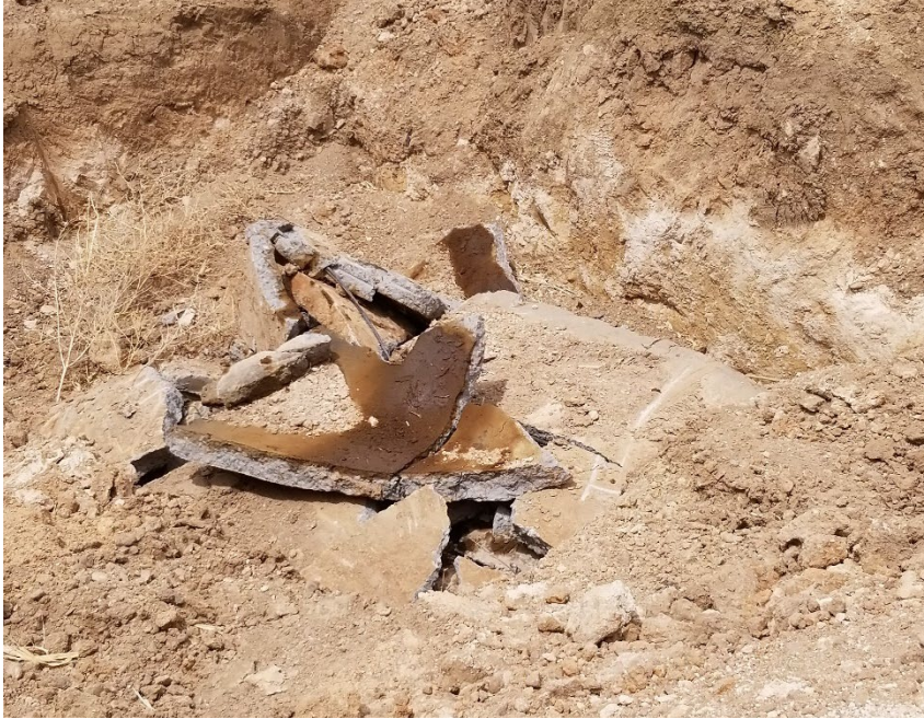
Concrete partially buried vessel, broken into pieces which were placed in an open excavation.
