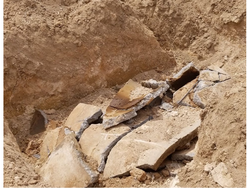
Concrete partially buried vessel, broken into pieces which were placed in an open excavation.
