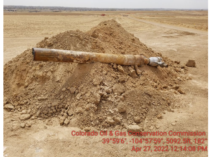
Spoils pile, and debris from cutting and capping the Sack G Unit 1, with inadequate stormwater BMPs.
