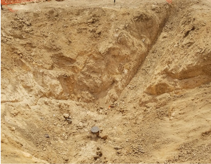
Sack G Unit 1 after being cut and capped.
