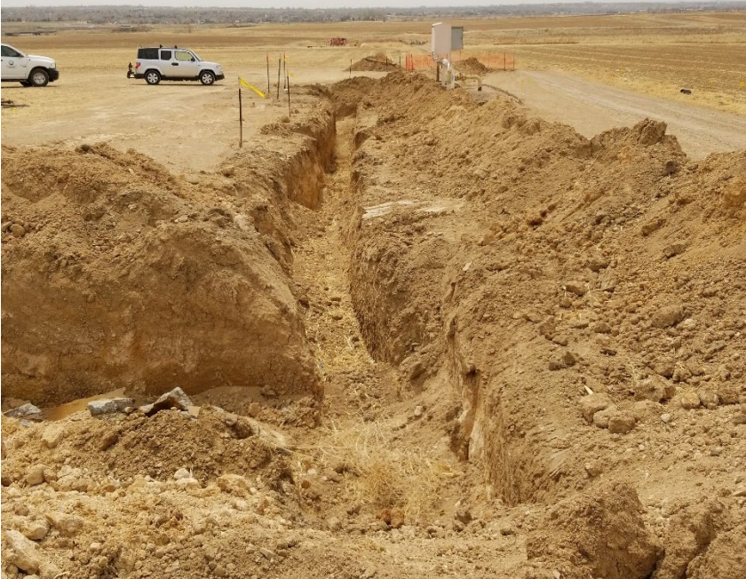
Open Excavation with inadequate safety fencing.
