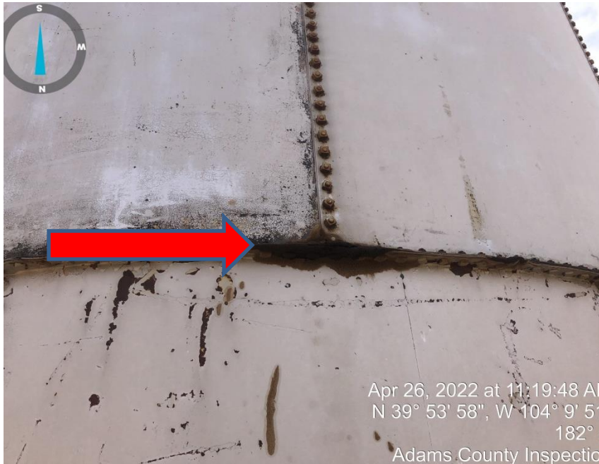
Photo#11 Small leak on north tank
