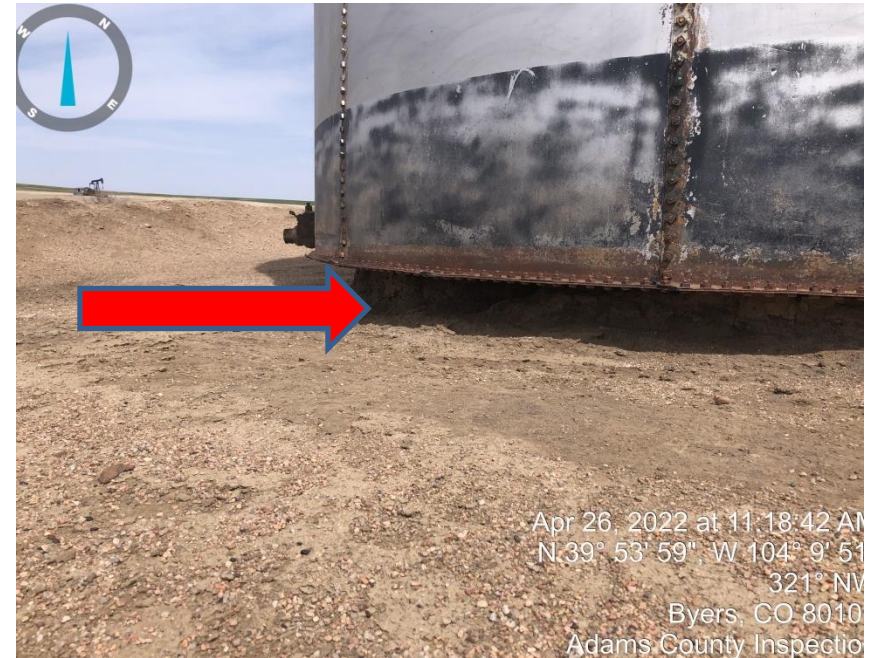
Photo#4 Large gaps under both production tanks
