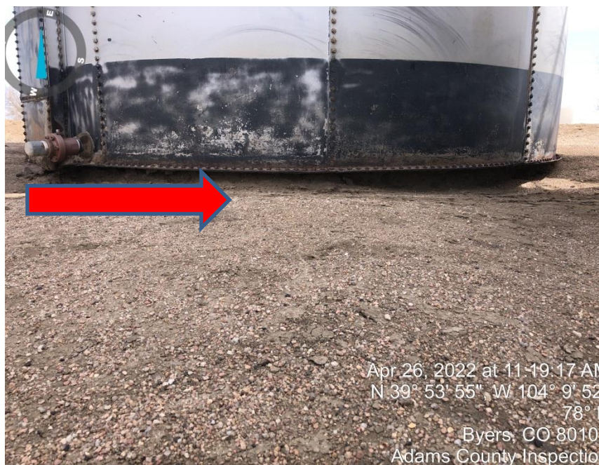
Photo#9 Large gaps under both production tanks
