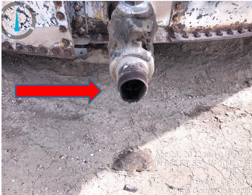
Photo#7 No Bullplug/Stained Soil
