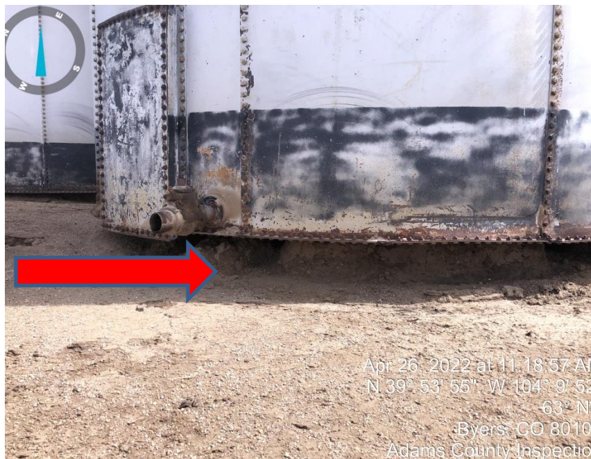
Photo#5 Large gaps under both production tanks
