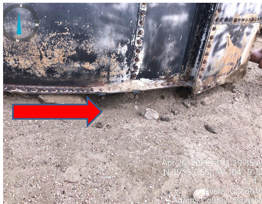
Photo#10 Large gaps under both production tanks
