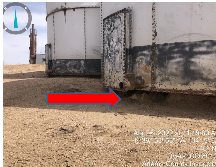
Photo#6 Large gaps under both production tanks
