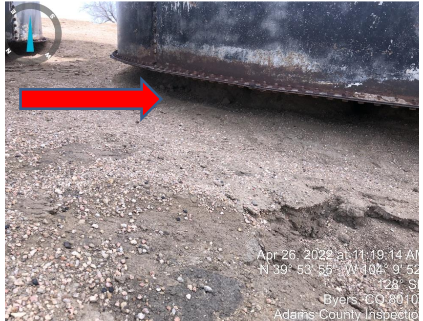
Photo#8 Large gaps under both production tanks
