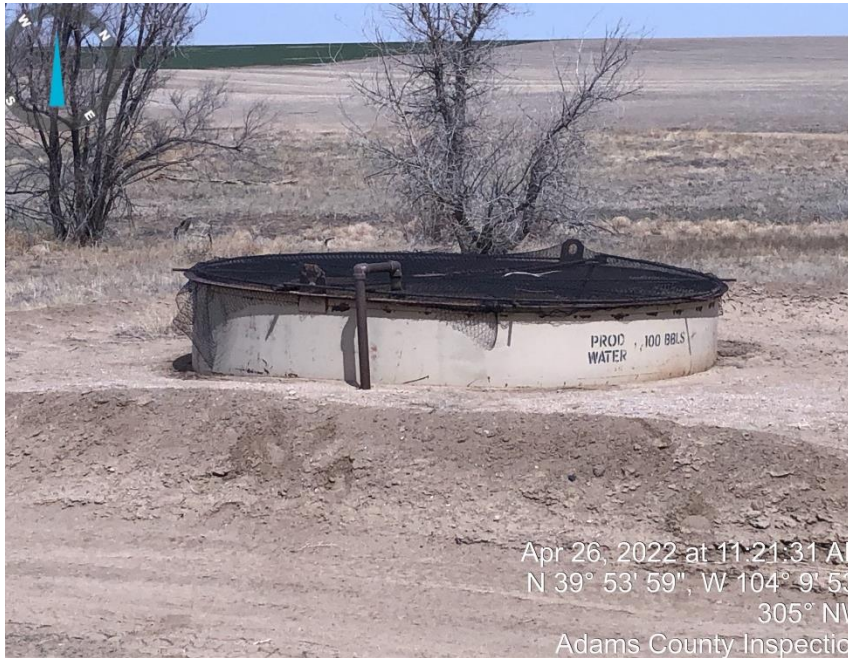
Photo#3 Produced Water Open Top Tank/Hydrocarbons in water. Open top tank is venting gas.
