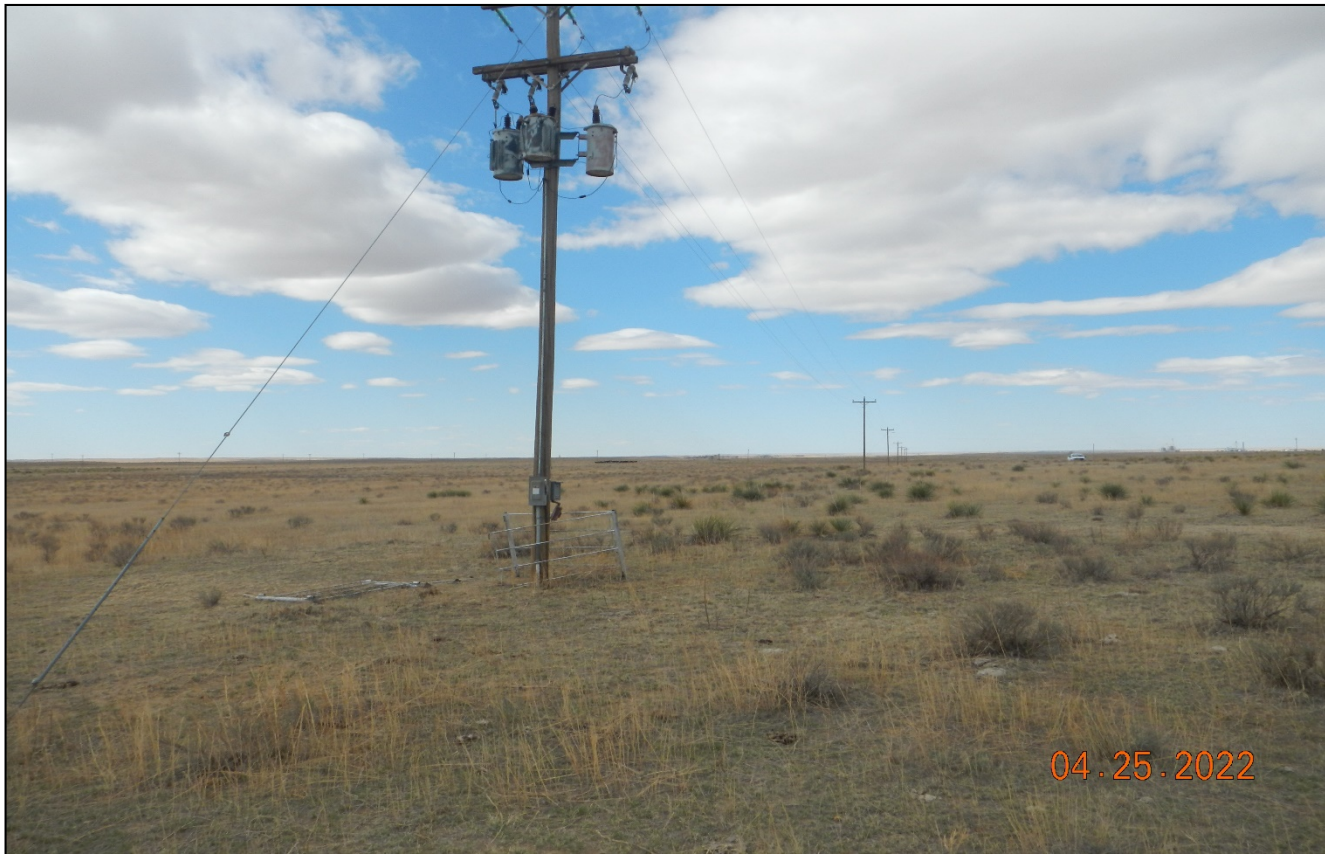
Photo 4. The powerline used for operating the well dead ends at the location and the entire unused portion of the powerline must be removed.
