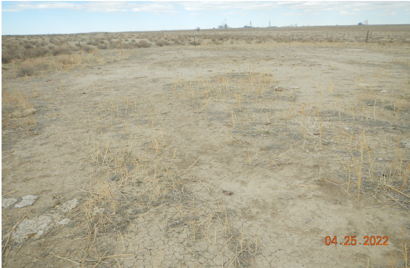
Photo 7. Facing northeast toward the abandoned well site. This area has not been reclaimed. Bare soils that are not stabilized and are susceptible to further erosion.
