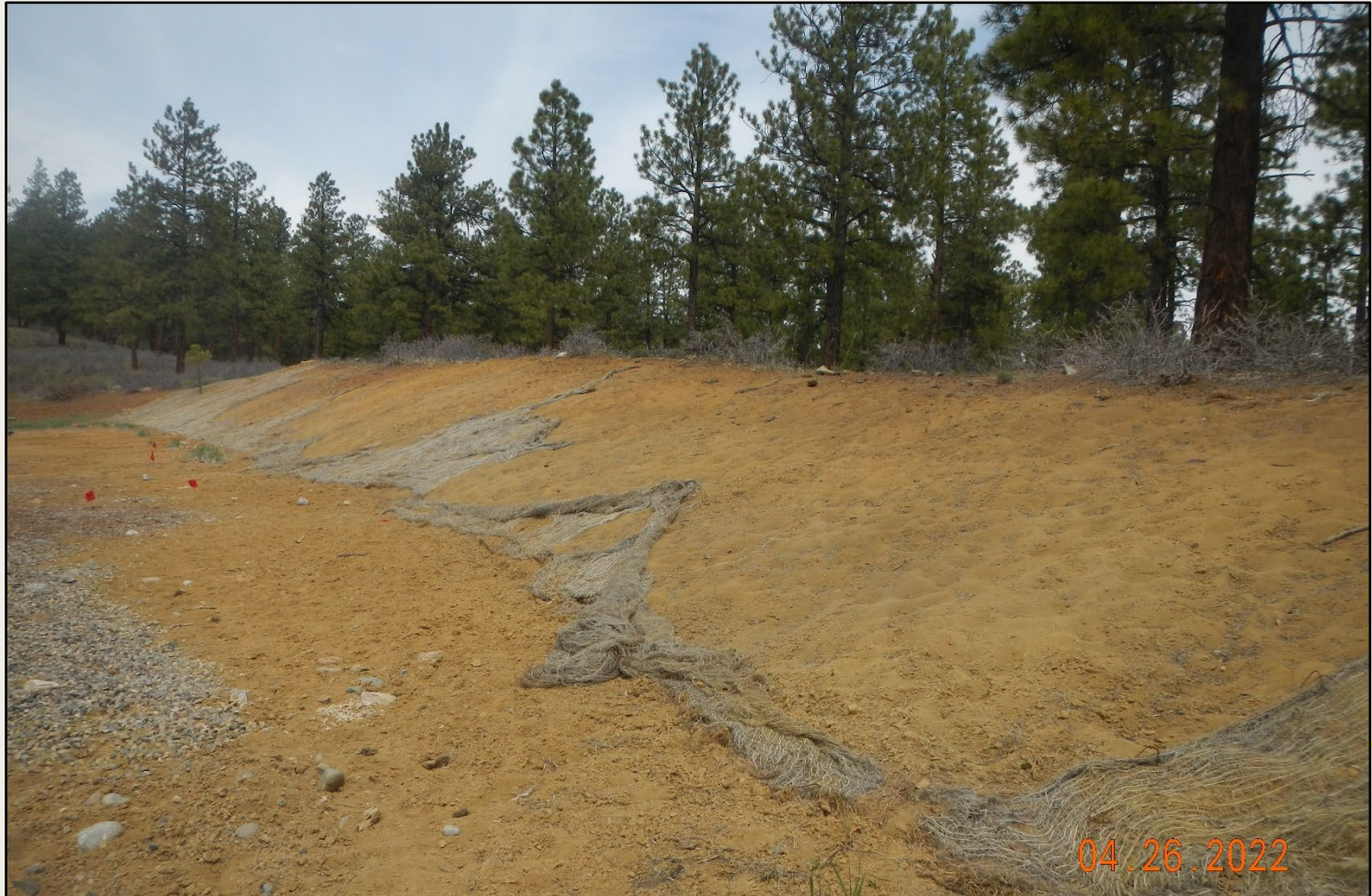
Photo 4. View of straw blankets on the well pad cut-slope no longer functioning.
