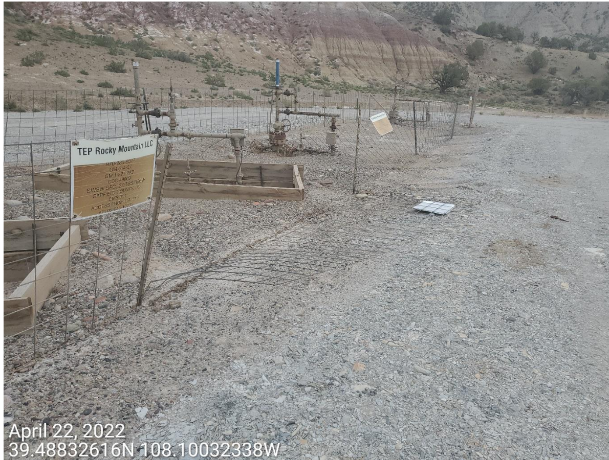
Photo 7: Photo shows fence panels at wells in disrepair.
