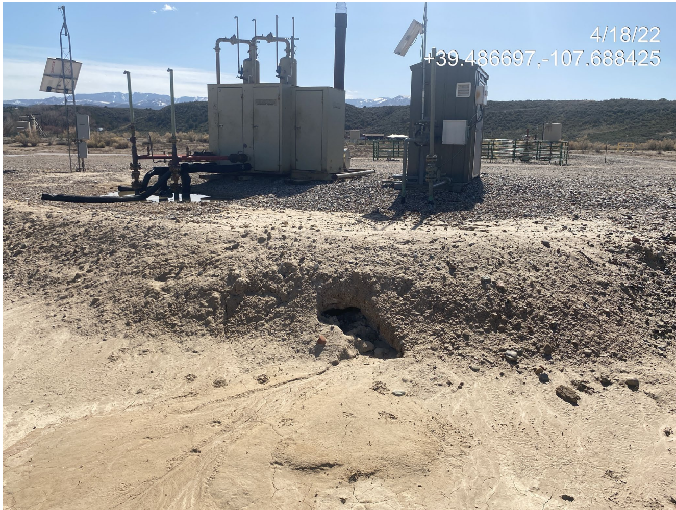
Photo 14. Photo taken from the east of the Location behind the separator shows the berm undermining. Sediment is coming through the berm.
