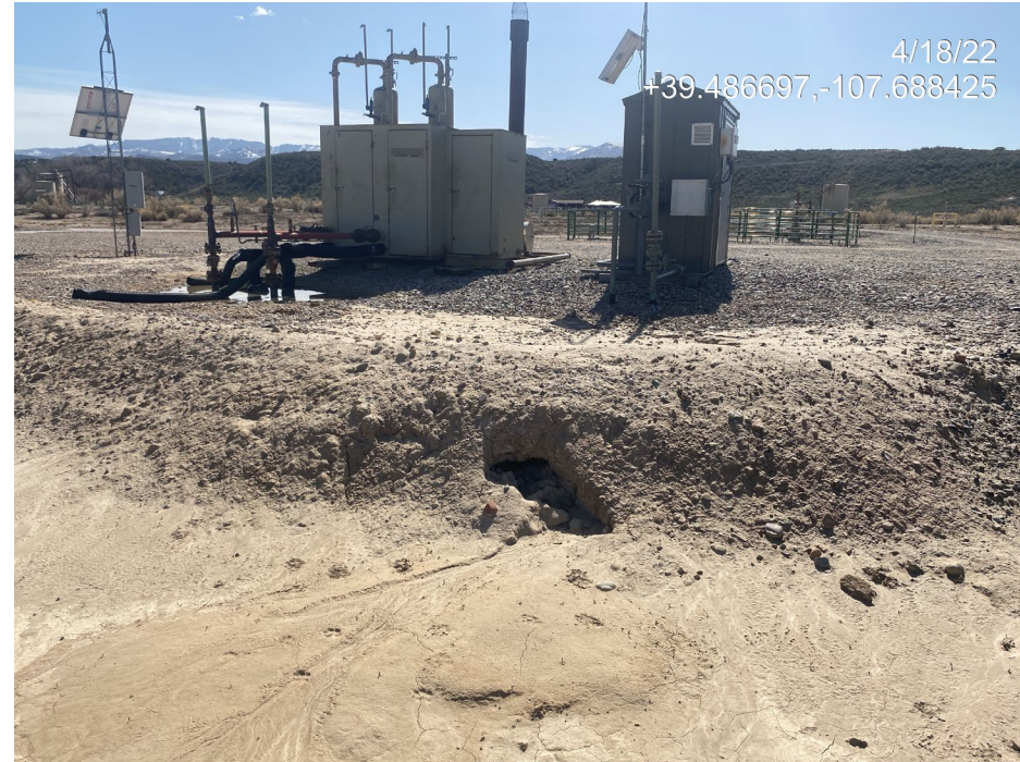
Photo 13. Photo taken from the east of the Location behind the separator. Photo is taken on the outside of the undermining berm where sediment is coming through.
