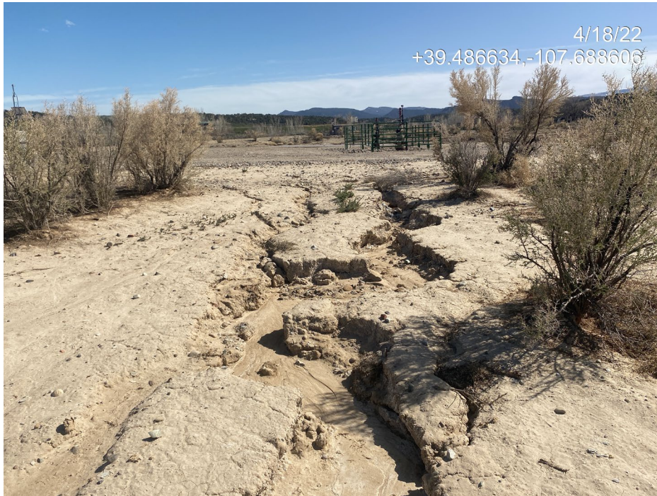
Photo 6. Photo taken from the north of the Location shows a gully developing on Location.
