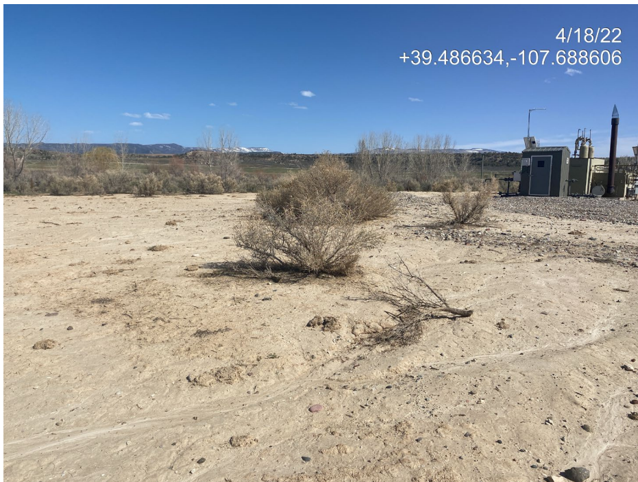
Photo 8. Photo taken from the north of the Location facing south shows erosion occurring in unvegetated/unstabilized interim areas.
