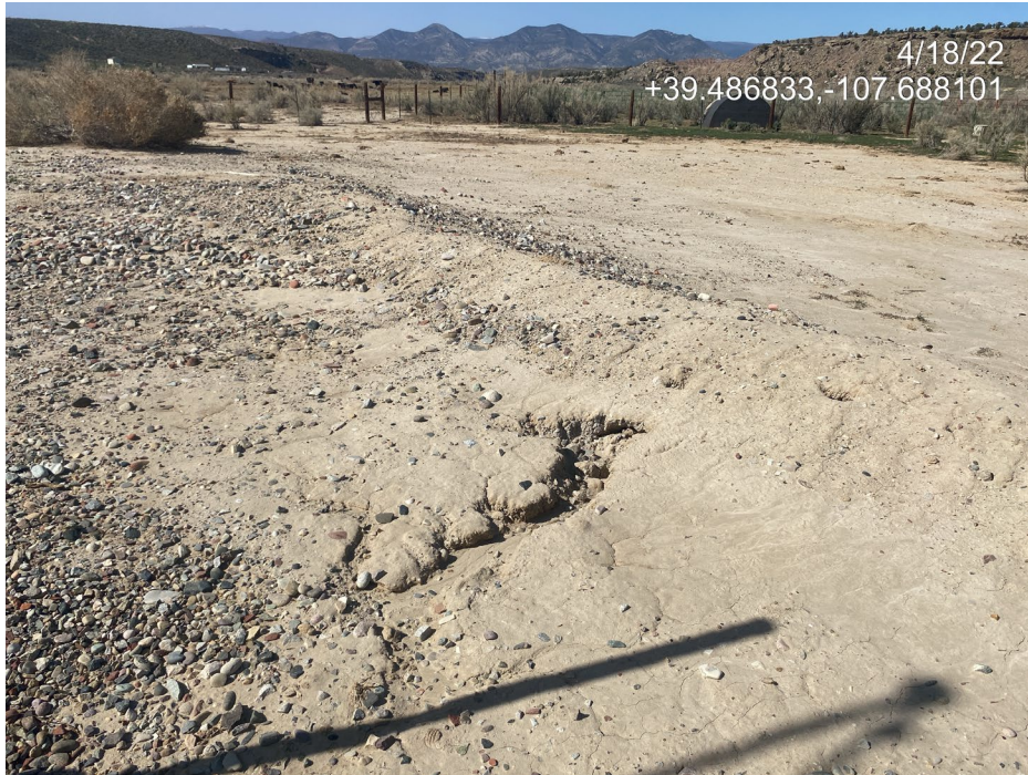
Photo 12. Photo taken from the east of the Location behind the separator. Photo is taken on the inside of the undermining berm where sediment is leaving the production area.
