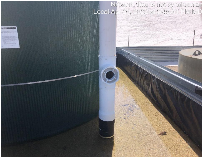
Photo #6533 Flowline heating insulation open ended.
