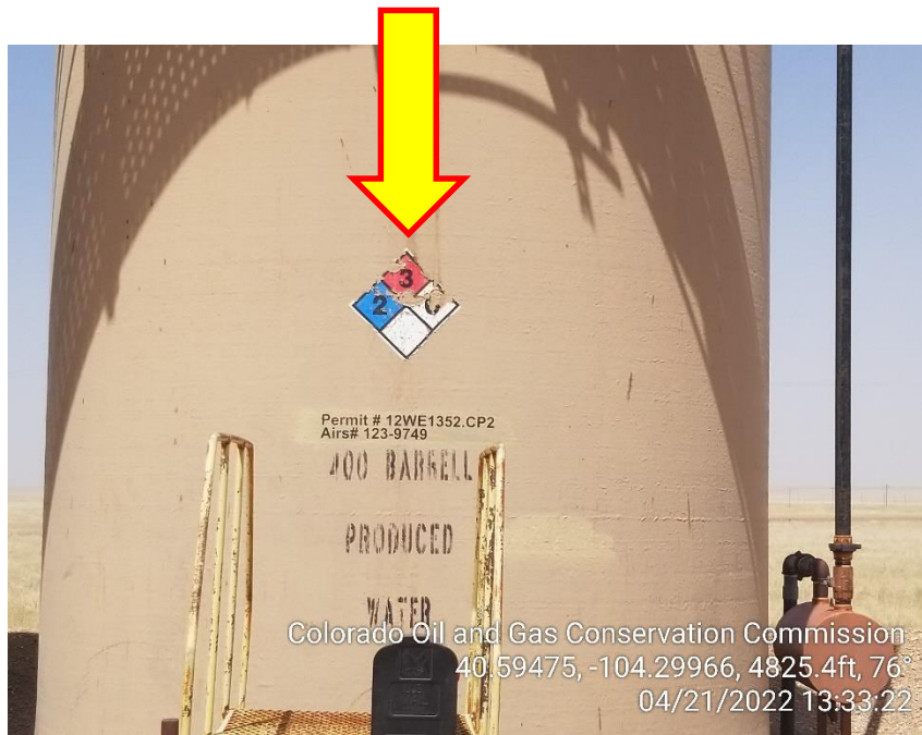
Photo 3 – NFPA Label has faded
