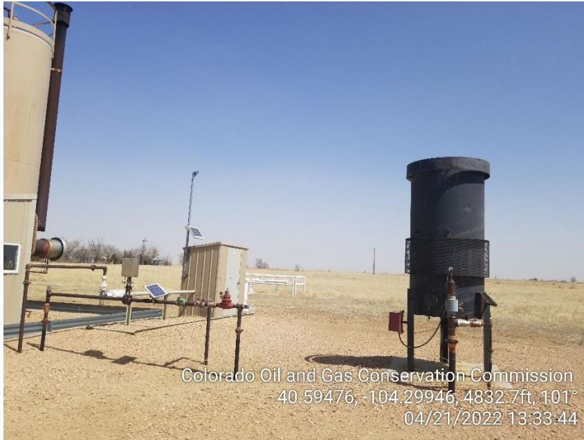
Photo 5 – ECD and Gas Meters
