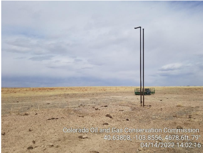
Photo 1 - Tank Flowline Risers
