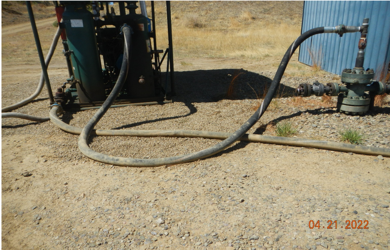
Photo 2. Facing toward the engine skid. Fluids were removed from the skid and gravel was placed around the skid but it does not seem stained soils were cleaned up.
