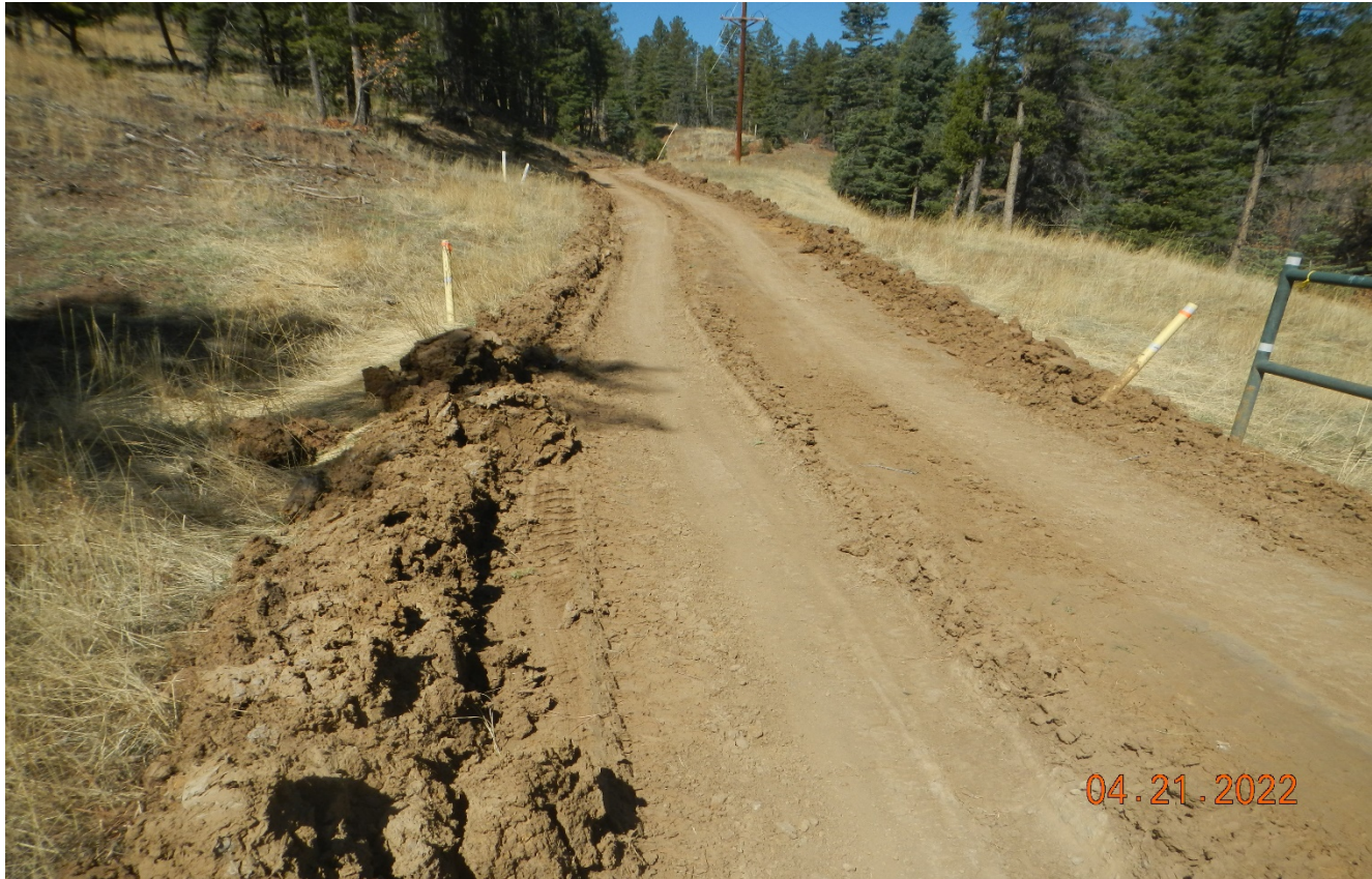
Photo 3. Facing west along the road. Soil material is graded off the road which will not allow drainage toward the culverts. The road is not stabilized and maintained.
