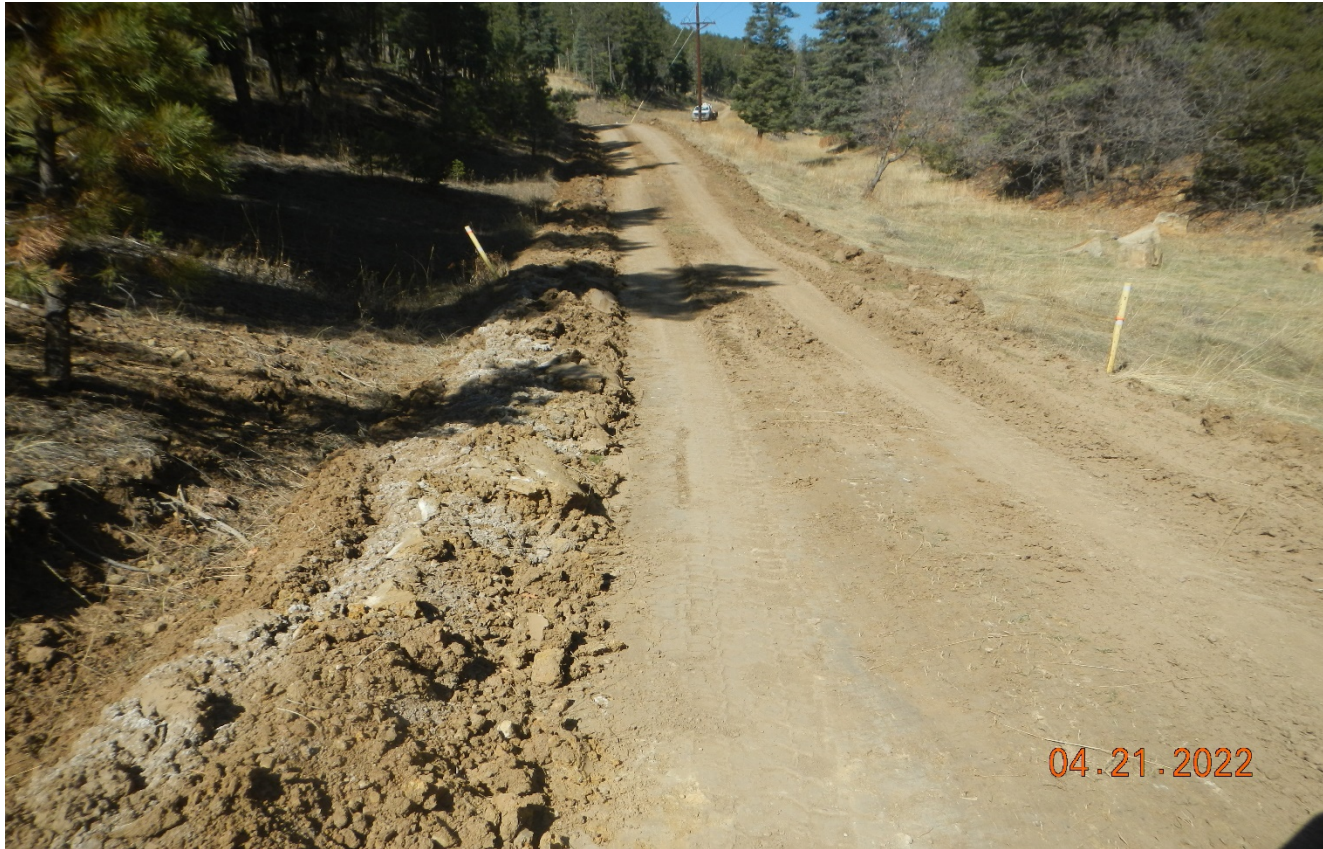
Photo 2. Facing west along the road. Soil material is graded off the road which will not allow drainage toward the culverts. The road is not stabilized and maintained.
