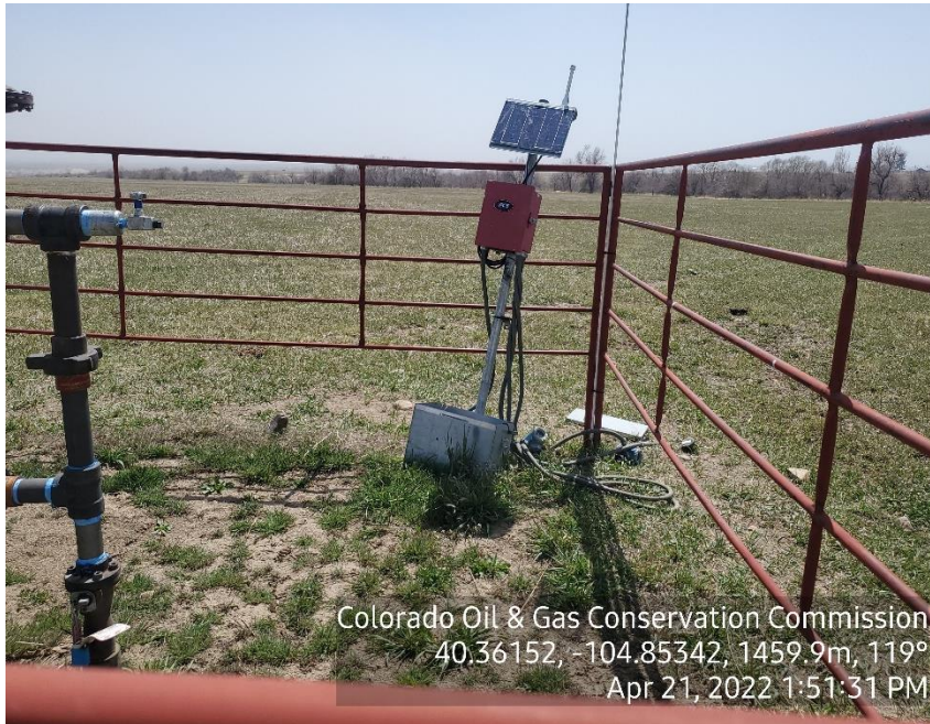
Photo 3: Disconnected automation
