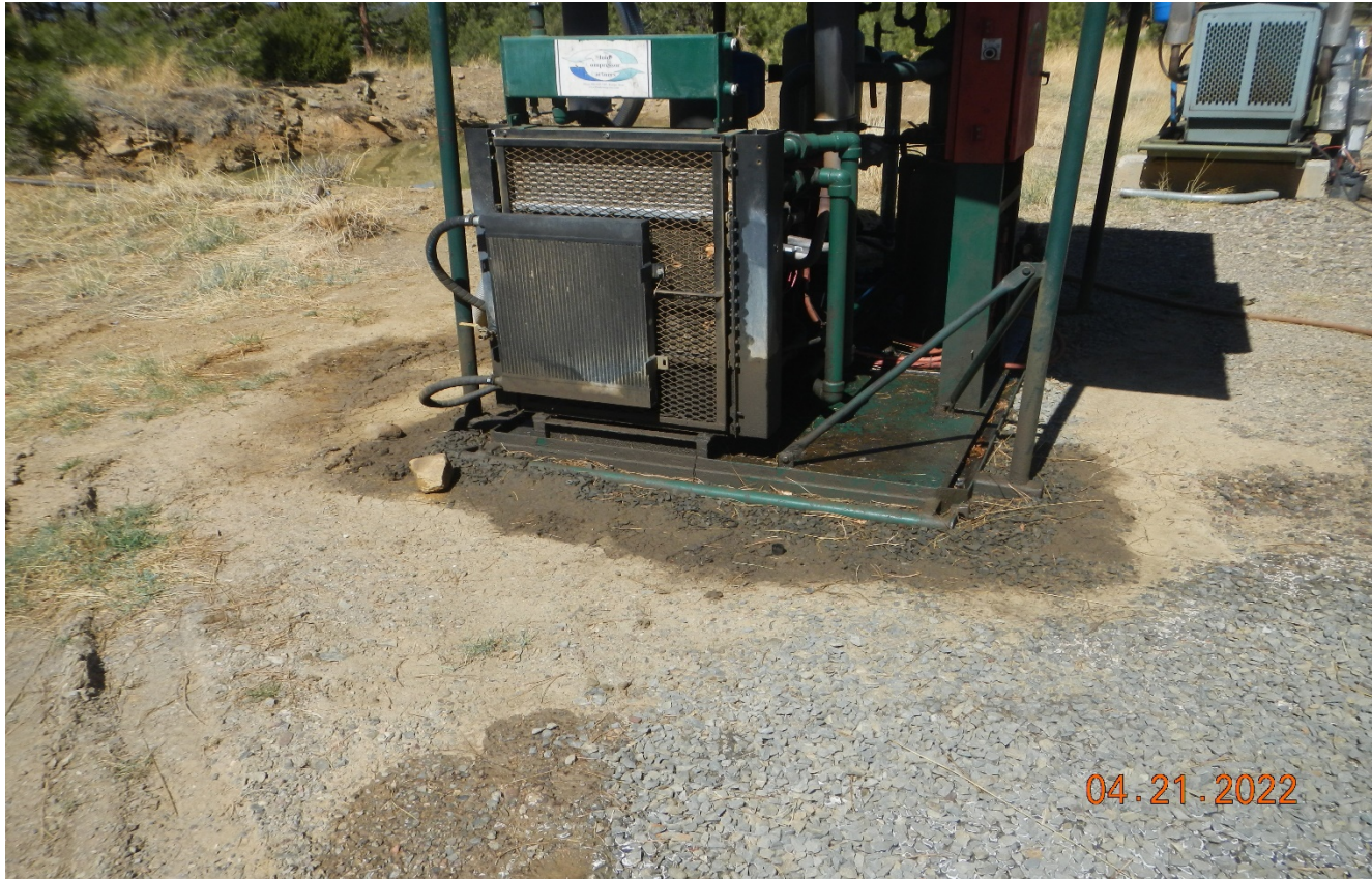
Photo 4. There is oil stained soils around the engine skid that needs to be cleaned up and properly disposed.
