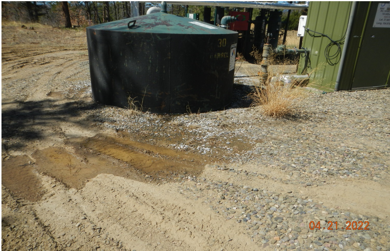
Photo 3. There is a dripping PW leak near the tank that needs repaired.
