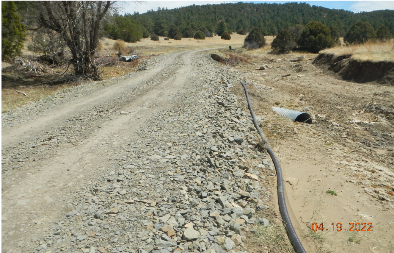
Photo 1. Facing southeast along the main access road. The black poly line remains exposed to potential damage.
