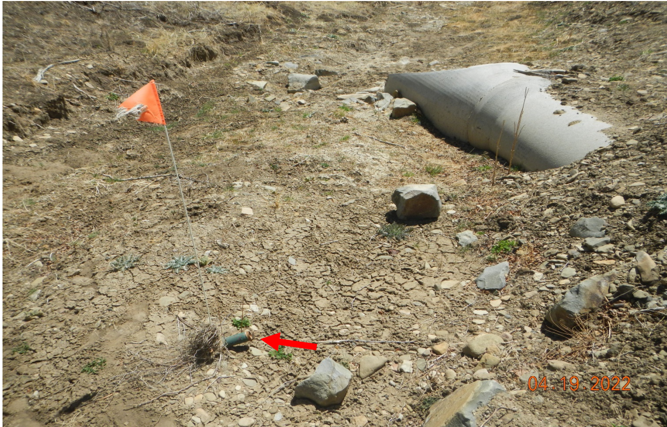
Photo 6. There is another produced water line that is bent over on the ground at the next crossing which needs to be repaired.
