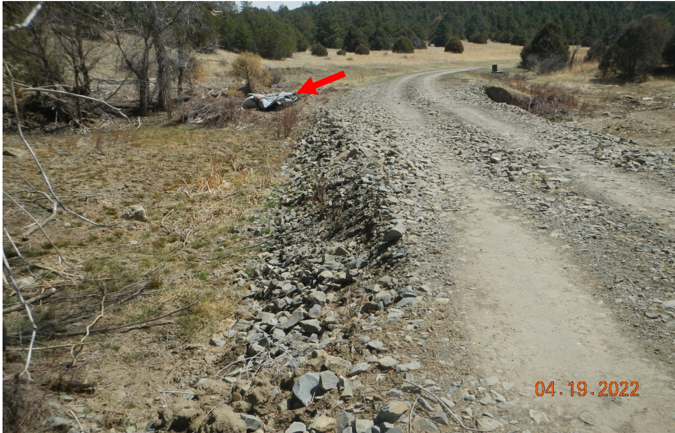
Photo 2. The damaged culvert debris needs to be removed.
