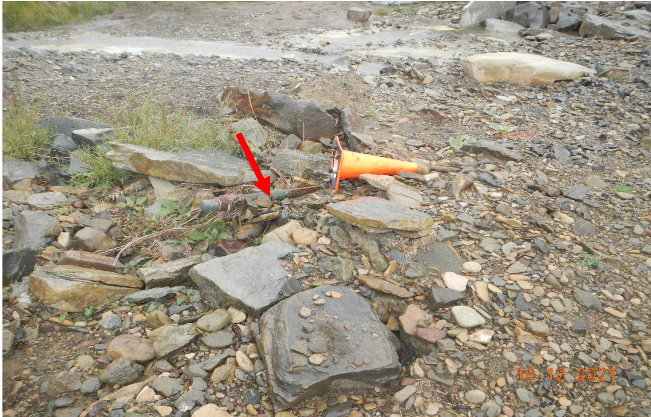
Photo 5. There is a produced water line that is bent over on the ground at the stream drainage which needs to be repaired. Previous corrective action was not completed. Photo taken from previous inspection but is also shown in previous photo.
