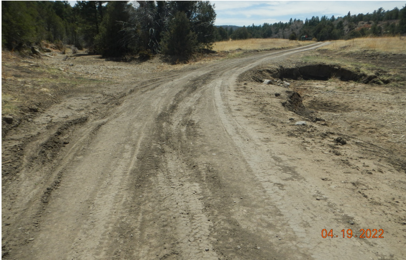
Photo 3. Facing south along the main road. The bank of the stream crossing needs to be stabilized. The cement culvert outlet should be reinstalled.
