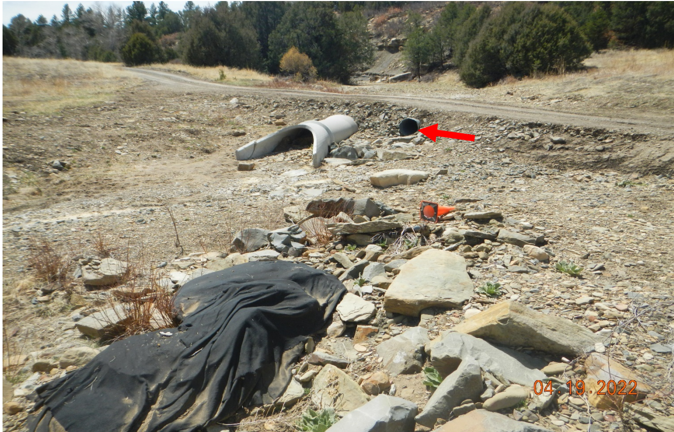
Photo 4. The cement culvert is filled in with sediment. The culvert at red arrow is not sufficient as shown by the size of the previous culvert. The liner debris in lower portion of photo needs to be removed. Previous corrective action was not completed.
