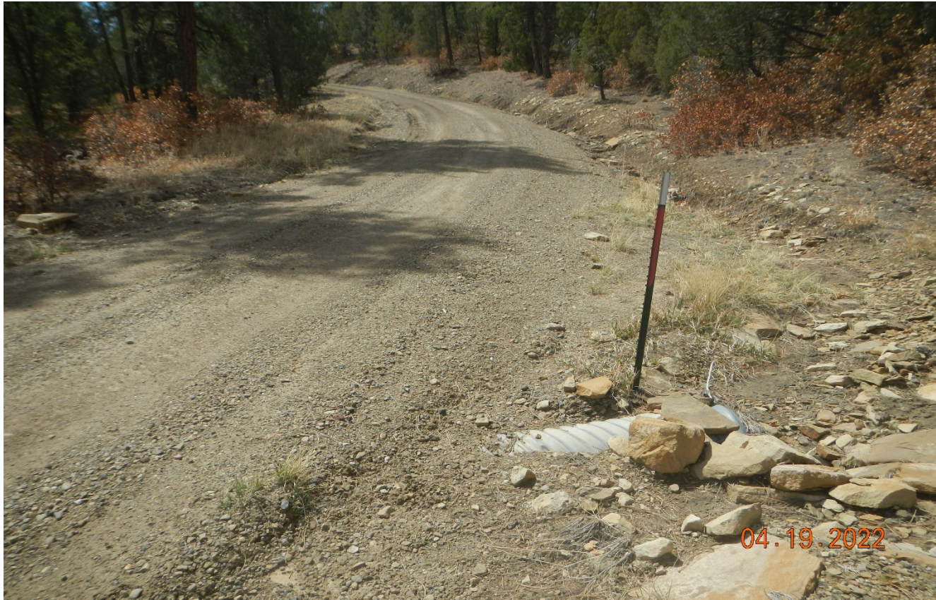
Photo 5. Another culvert further along the road is filled in with sediment.
