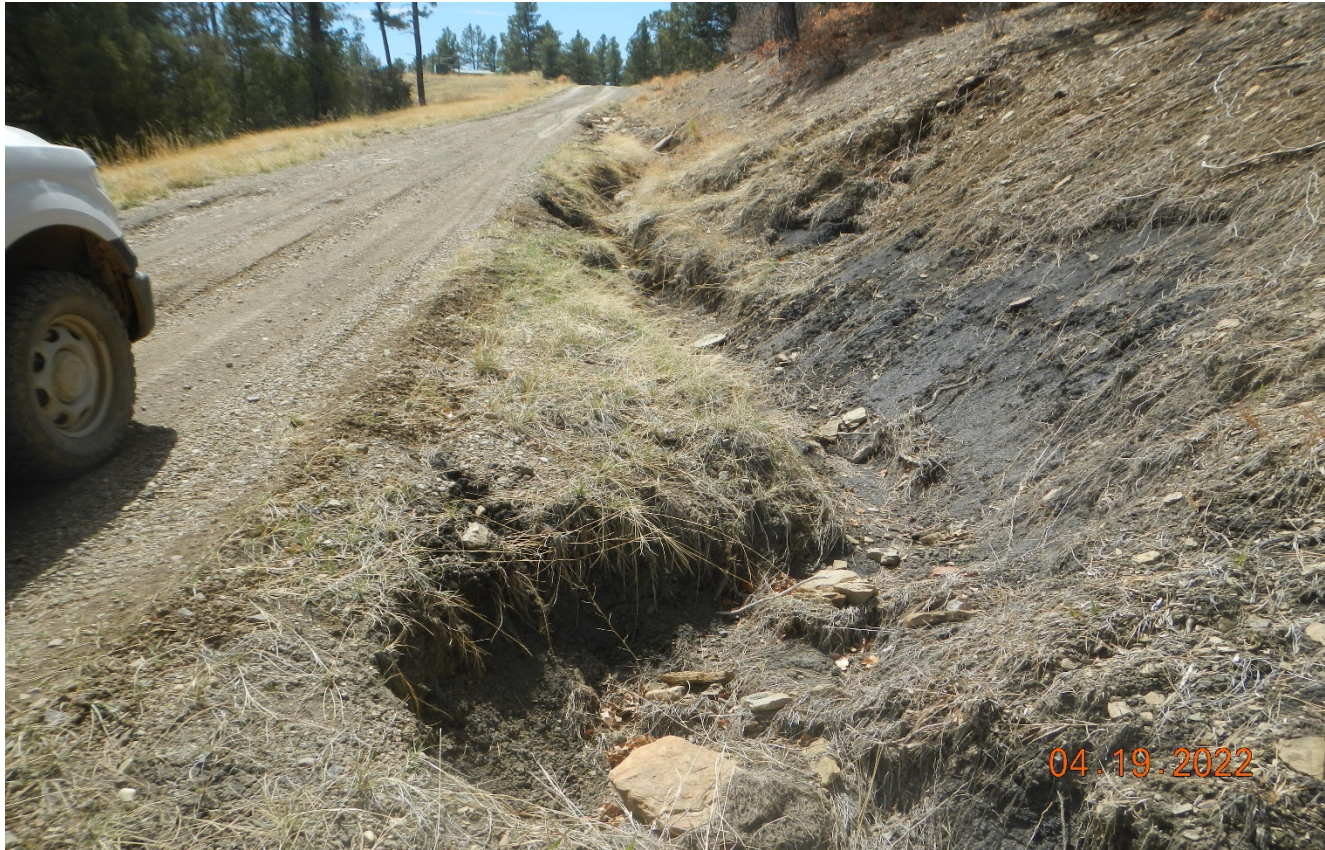
Photo 7. Facing southeast along the access road near the location. Erosion along the roadside has exposed a pipeline in this area.
