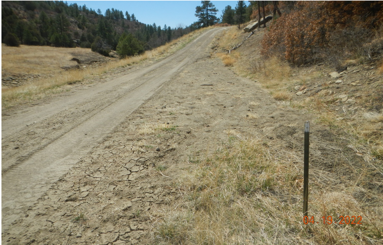
Photo 3. Facing southeast along the access road. The culverts along the access road are filled in with sediment.
