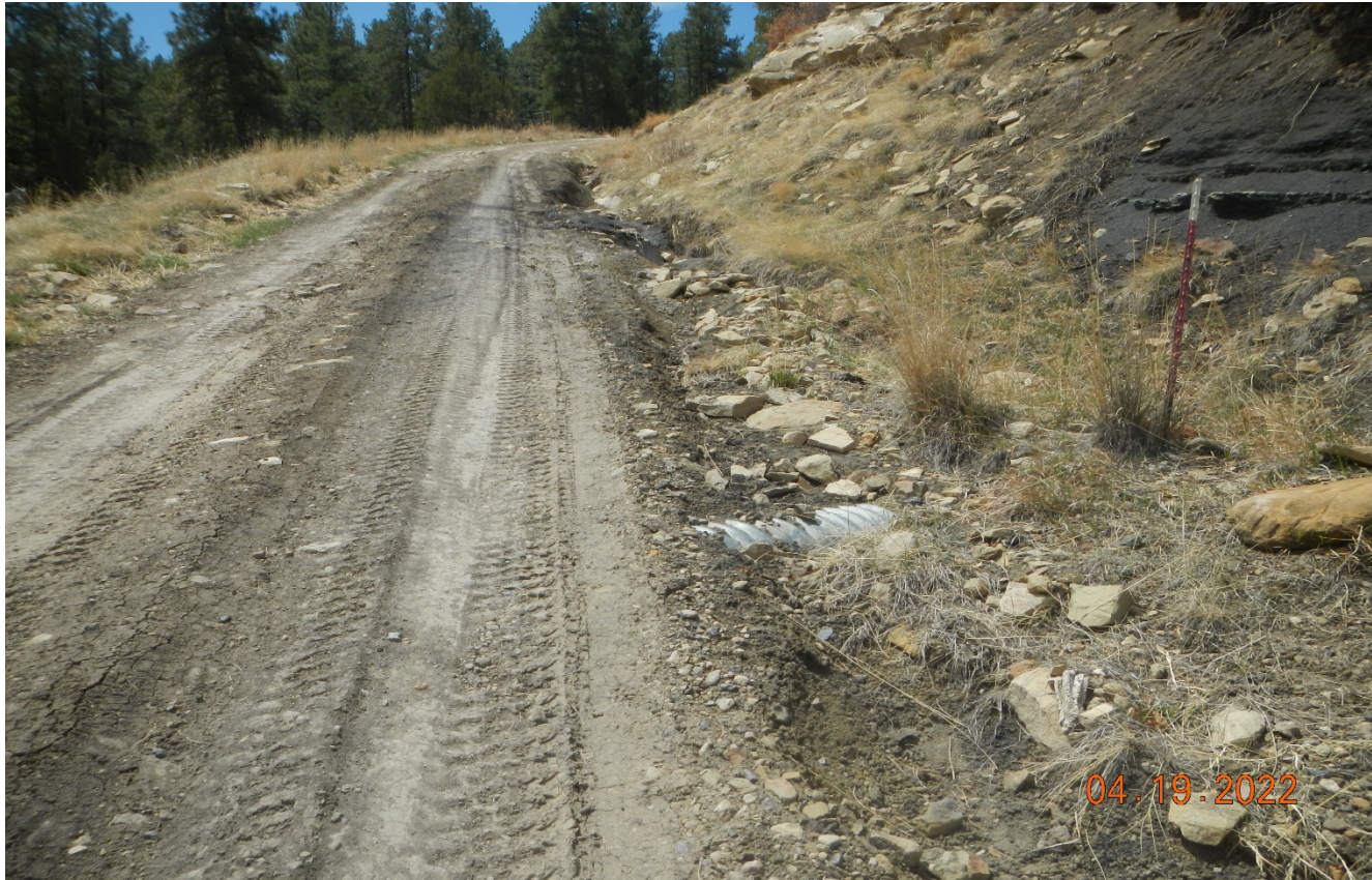
Photo 4. The culverts along the access road are filled in with sediment causing stormwater erosion down the road.
