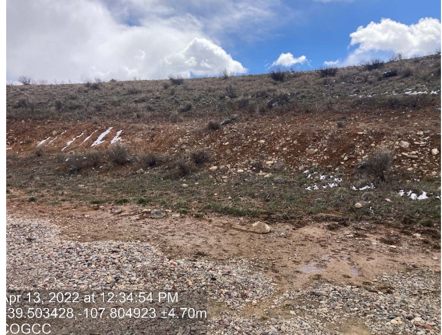
Cut slope shows signs of lack of stabilization/ erosion
