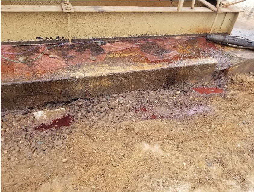
Photo 7. Free fluid in spill at pump jack.
