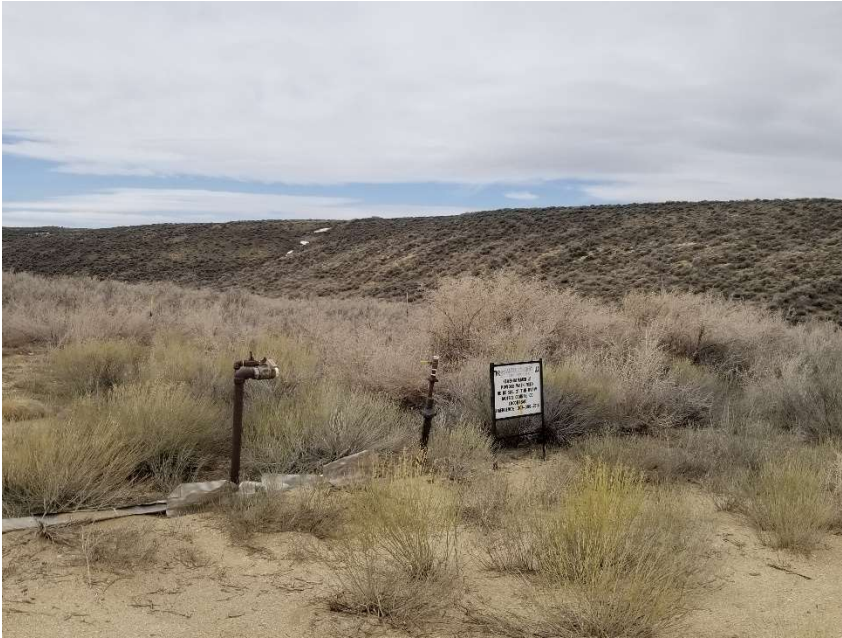
Photo 3. Unmarked risers at wellhead.
