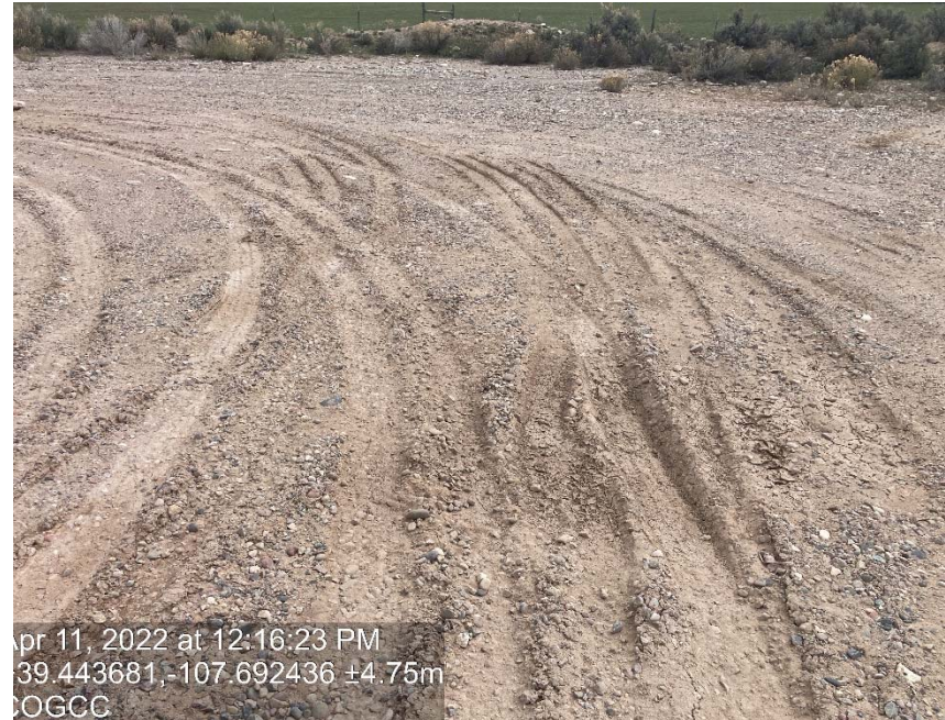
Some areas of lack of stabilization/compaction
