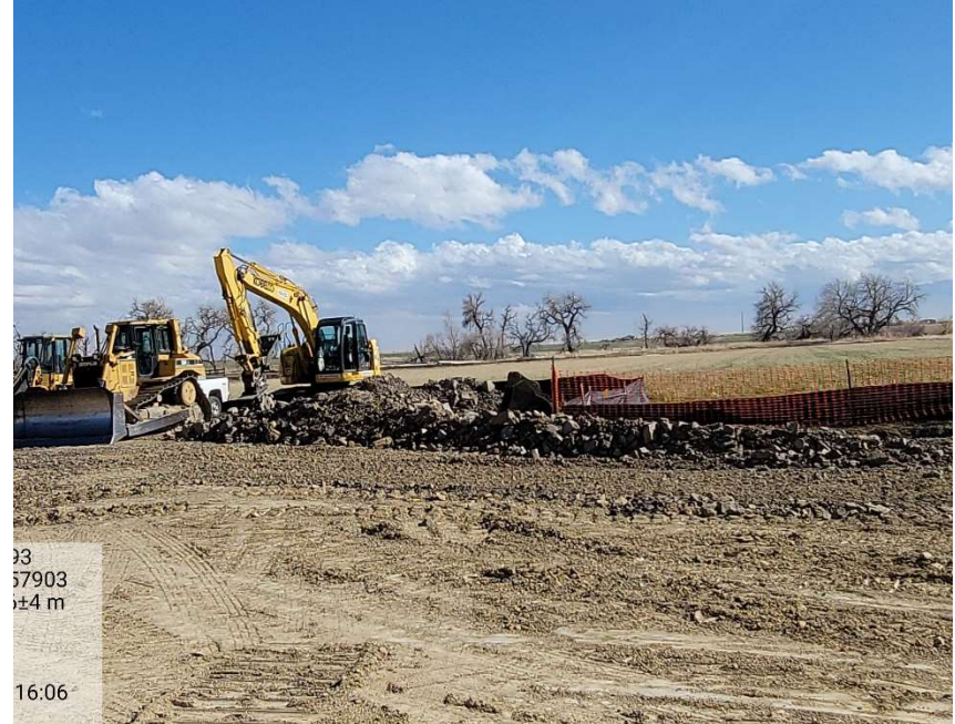
Photo 8 – April 5, 2022 – Stockpiled soil with inadequate BMPs
