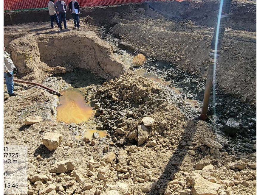
Photo 4 – April 5, 2022 – Initial spill response to new spill: Hydrovac
