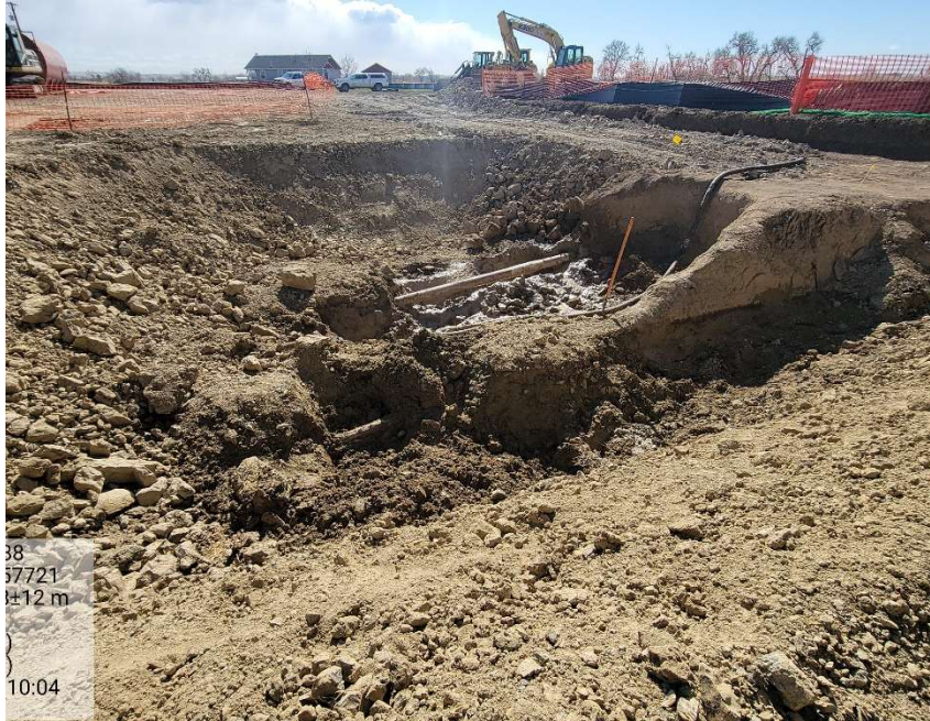
Photo 9 – April 7, 2022 – Fencing and exposed flowline
