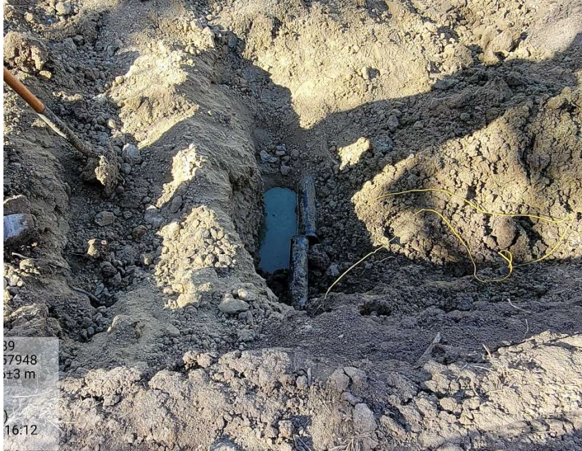
Photo 3 – April 5, 2022 – Initial spill response to new spill: Exposed damaged flowline
