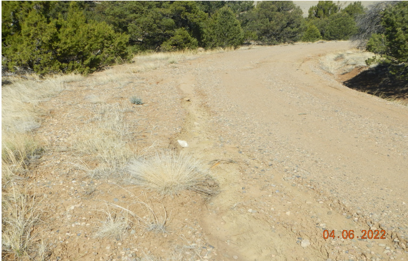
Photo 1. Facing northwest along the access road. There is an erosion channel along the road that needs to be repaired and stabilized.
