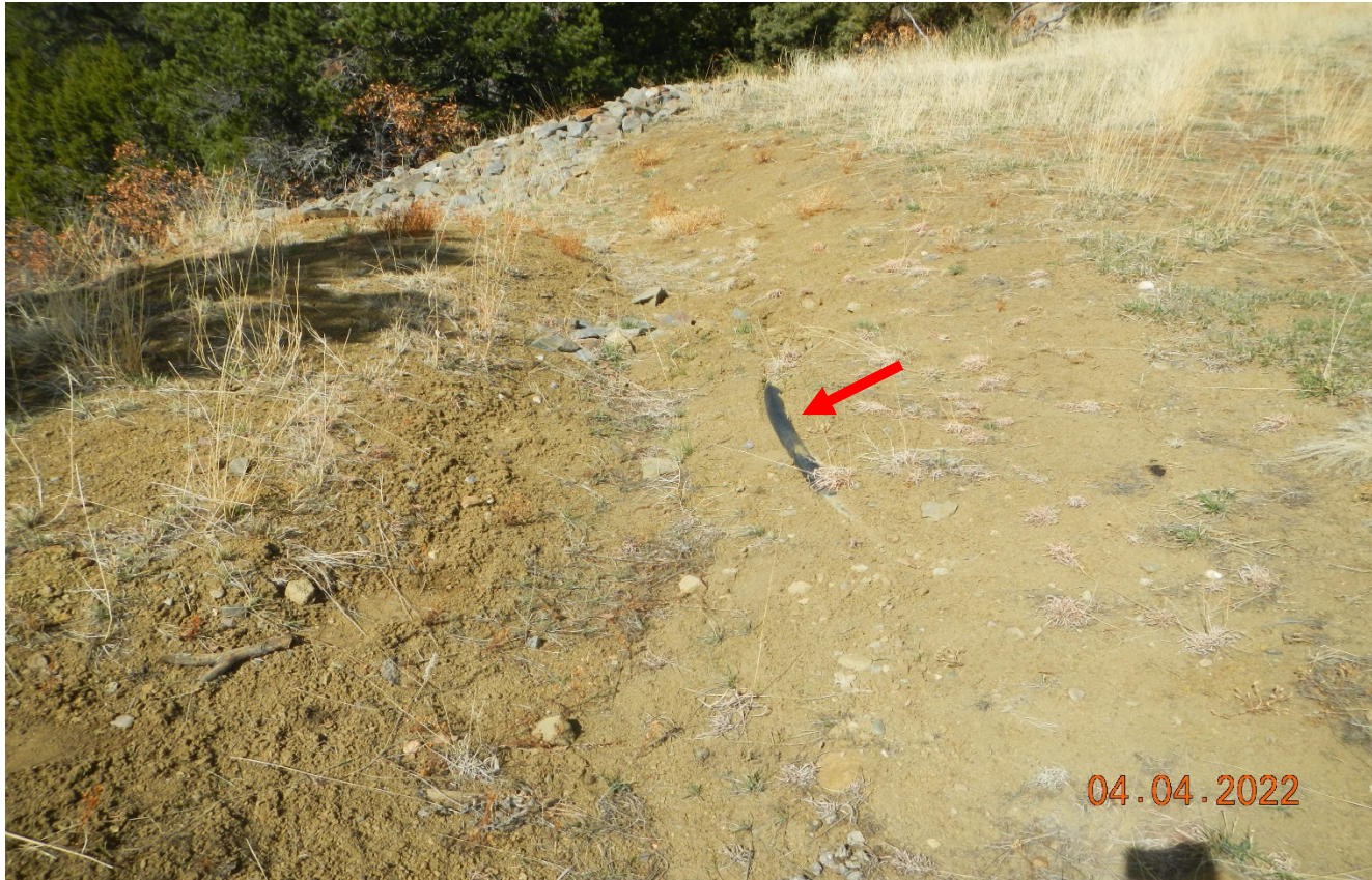
Photo 9. There is a exposed black poly line at the southwest side of the location.
