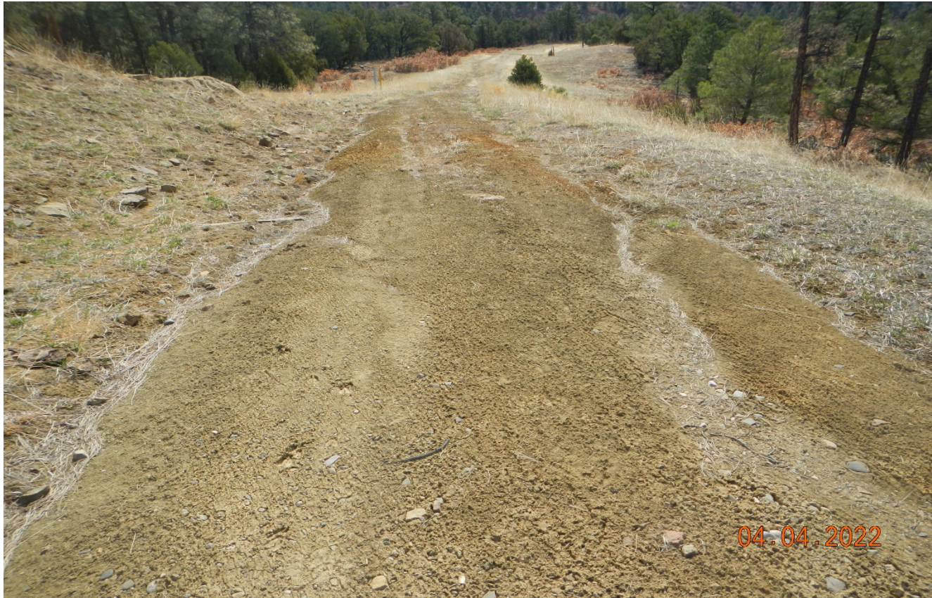
Photo 2. Facing southeast along the road. There are signs of erosion in this area of the road.
