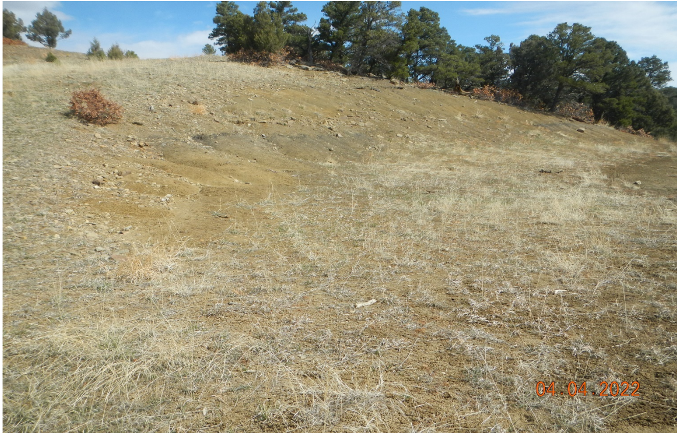
Photo 4. Facing toward the cut slope. There are signs of erosion along the cut slope which is not stabilized.
