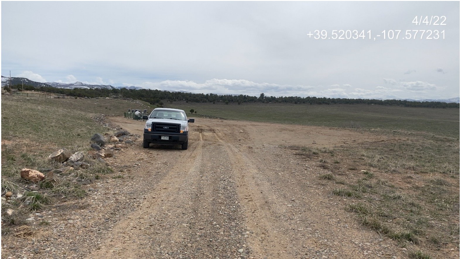
Photo 2. Photo taken from the Location entrance facing south shows an overview of the Location and the lack of stabilization BMPs as is evidenced by the presence of ruts.
