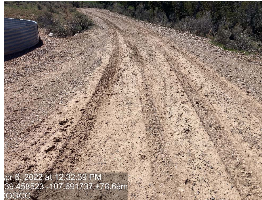
Access road in areas show signs of lack of stabilization
