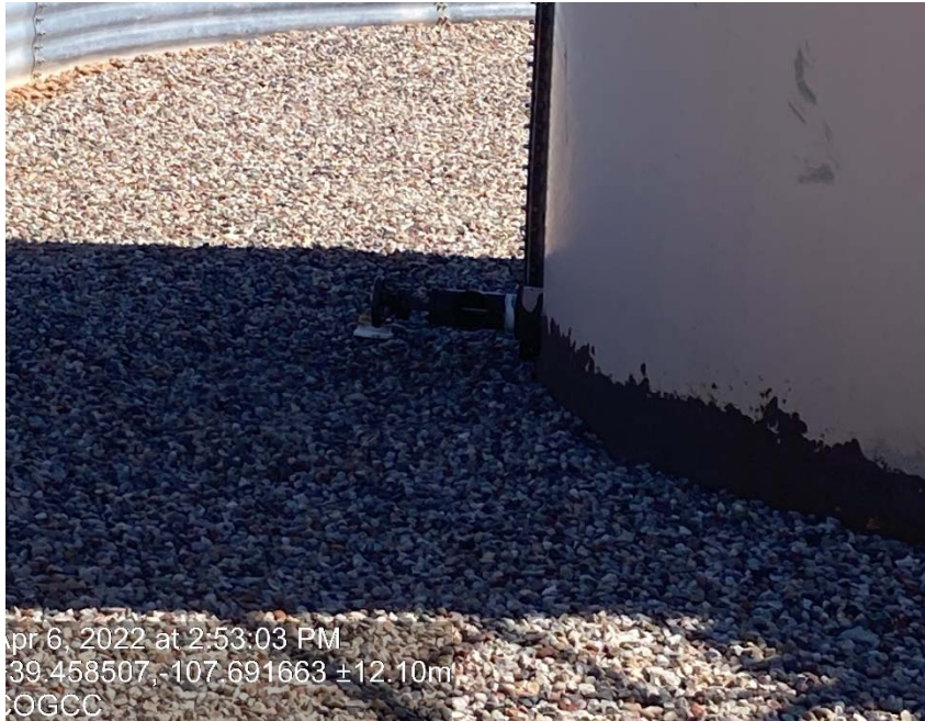
Line on tank missing cap/plug
