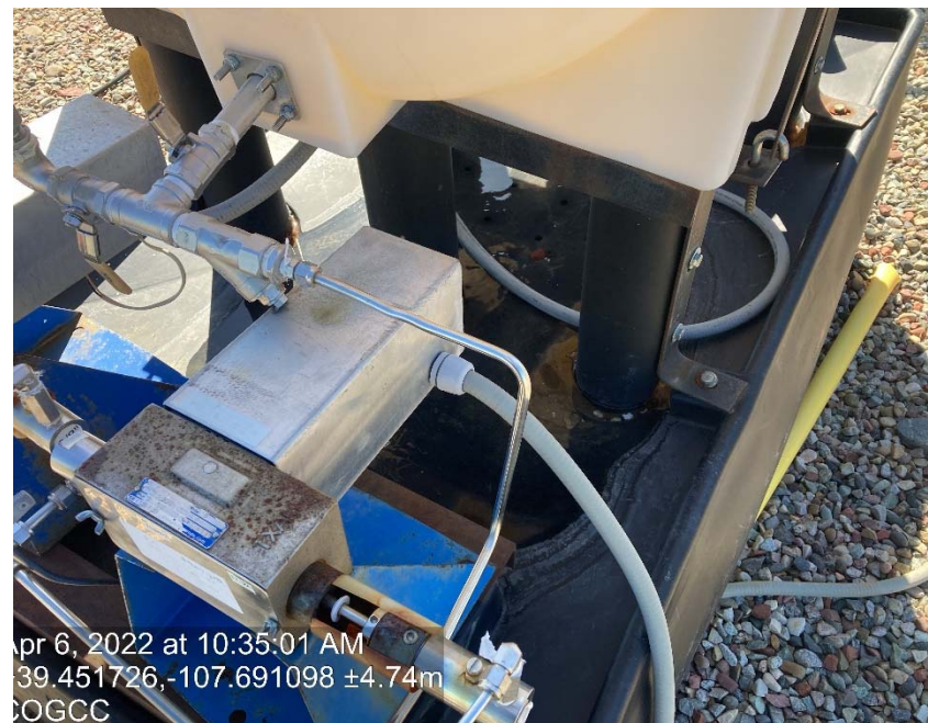
Chemical tank containment is full of fluid
