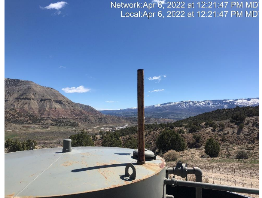
Photo #6372 Vent pipe on tank open ended.
