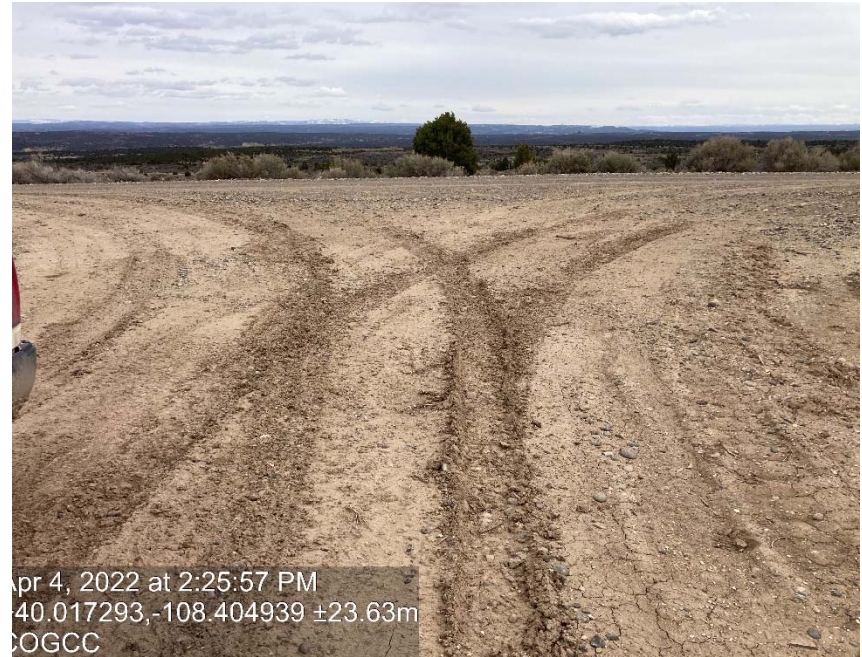
Location/ lack of stabilization/compaction
