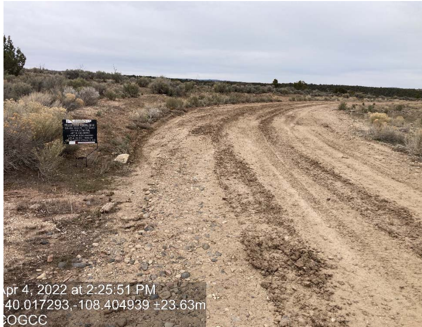
Location/ lack of stabilization/compaction
