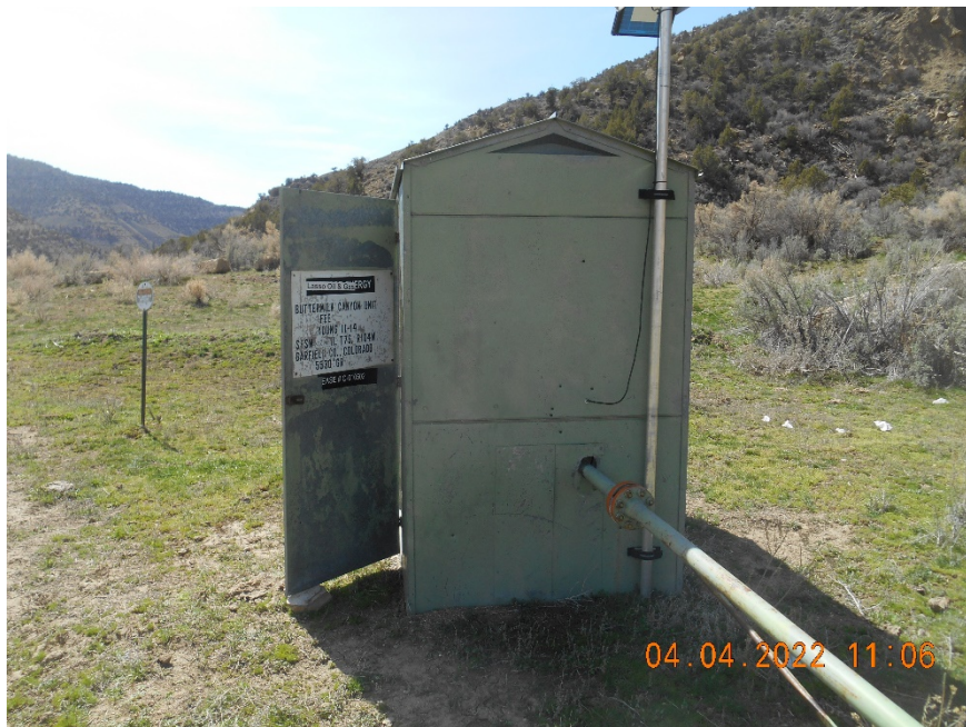
Separator and Meter Housing with sign
