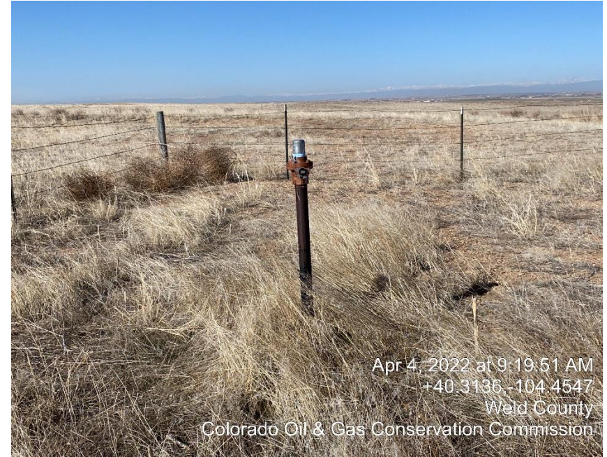
Photo #2 Unmarked Riser
