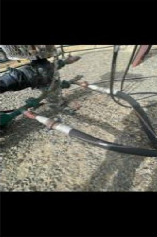
Conducted Maintenance on equipment (Repaired Leaks), cleaned up stained material and reviewed self-inspection to comply with Rule 1002,.(2)D.
