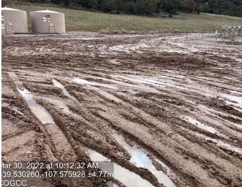
Lack of stabilization/ compaction/ degradation
