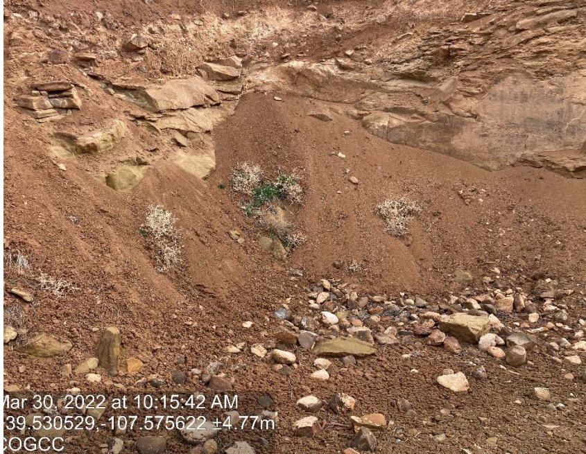
Cut slope erosion
