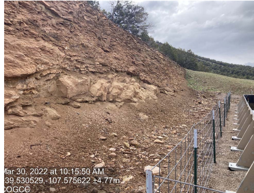
Cut slope erosion/ lack of stabilization
