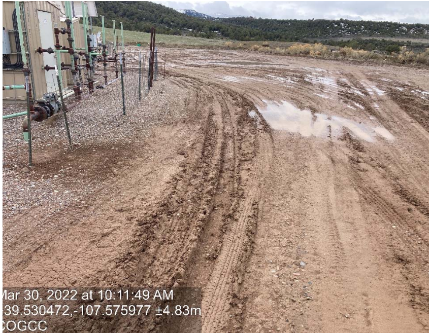
Lack of stabilization/ compaction/ degradation
