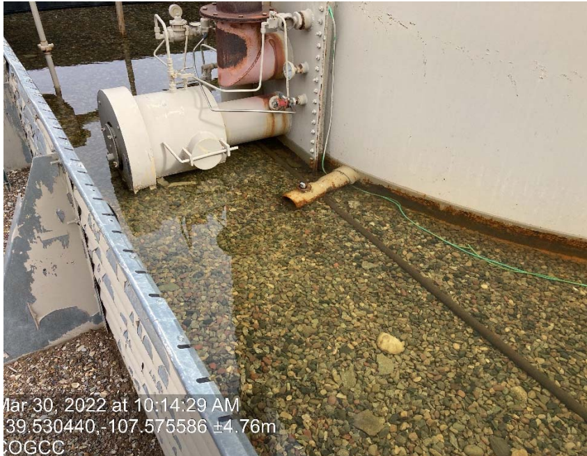
Valve missing cap/plug under water
