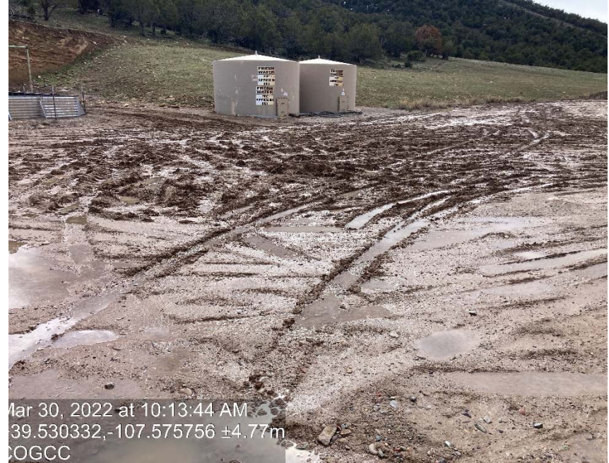
Lack of stabilization/ compaction/ degradation
