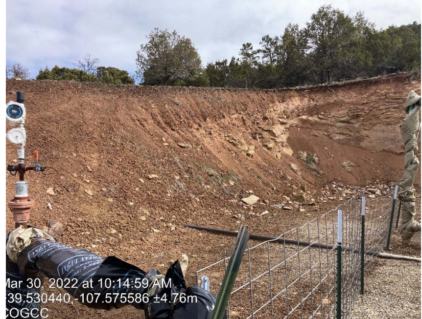
Cut slope erosion/ lack of stabilization
