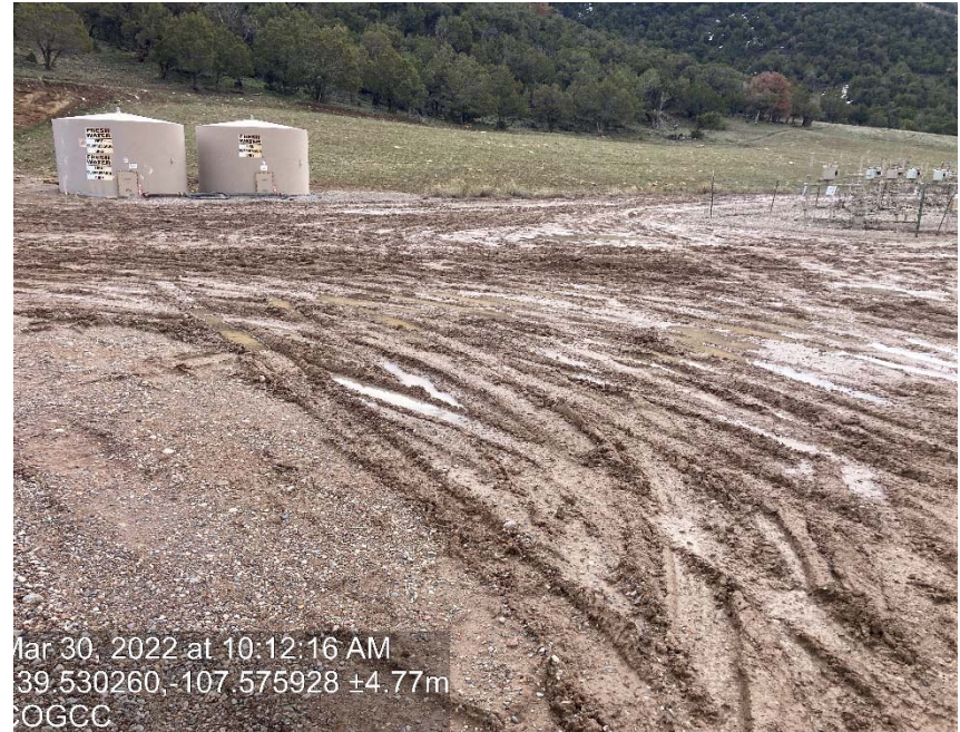
Lack of stabilization/ compaction/ degradation
