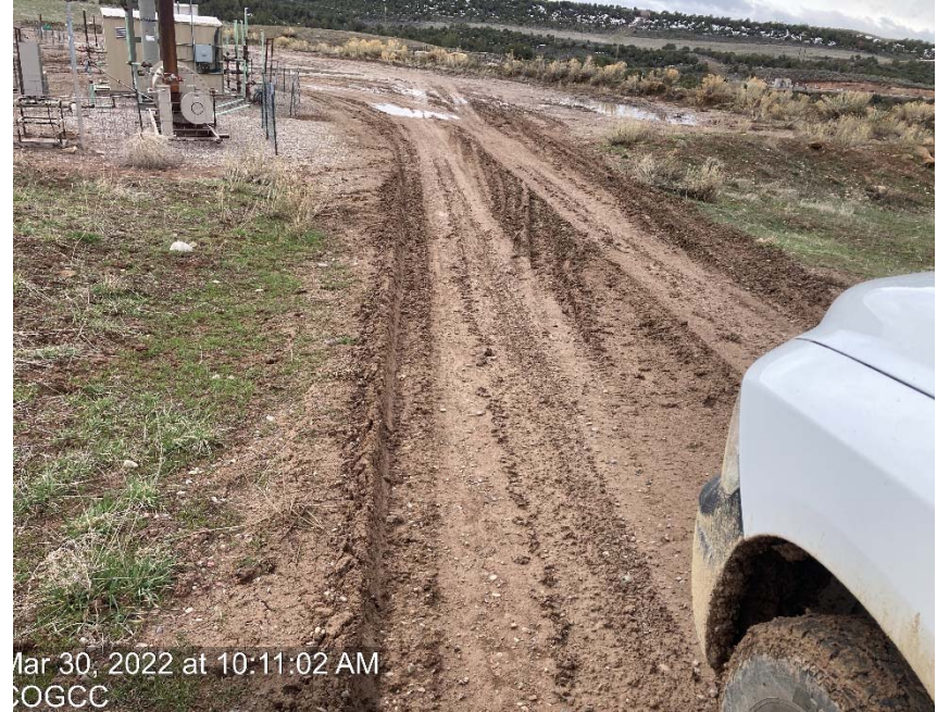
Lack of stabilization/ compaction/ degradation
