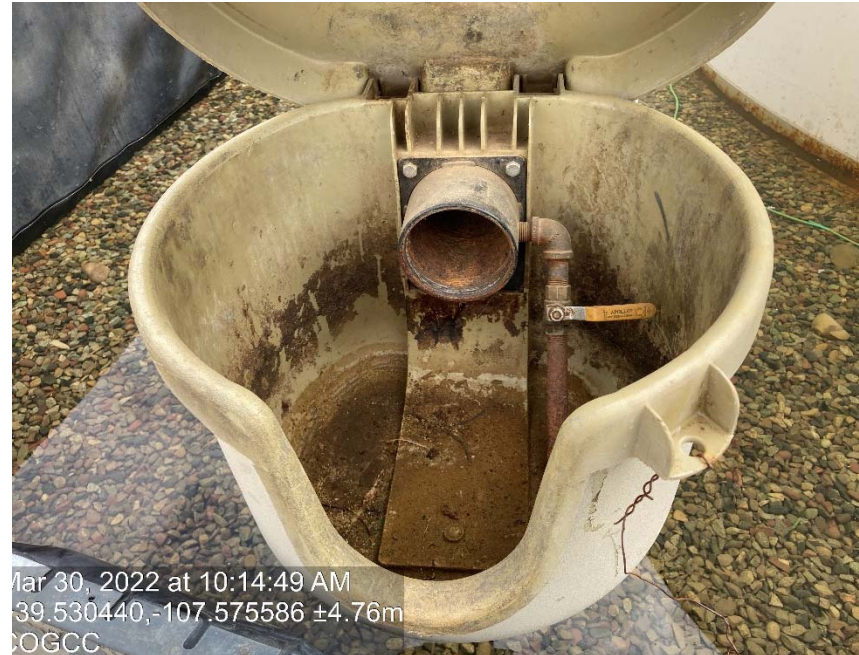
Valve missing cap/plug
