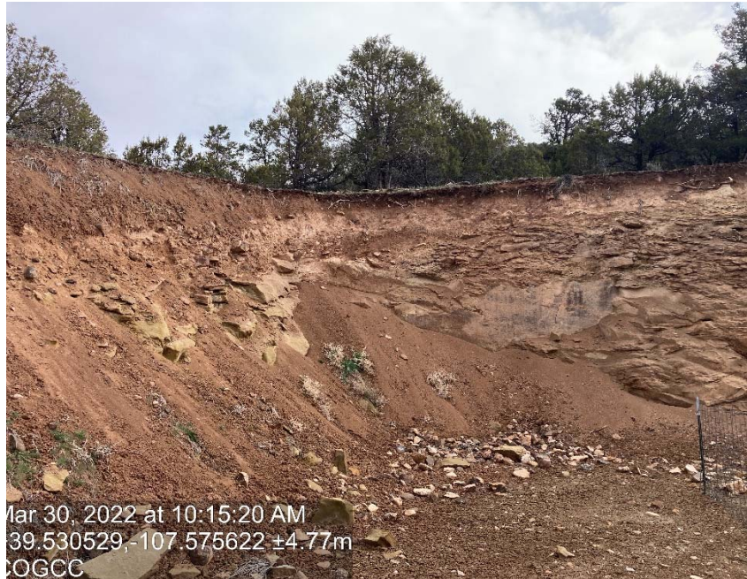
Cut slope erosion/ lack of stabilization
