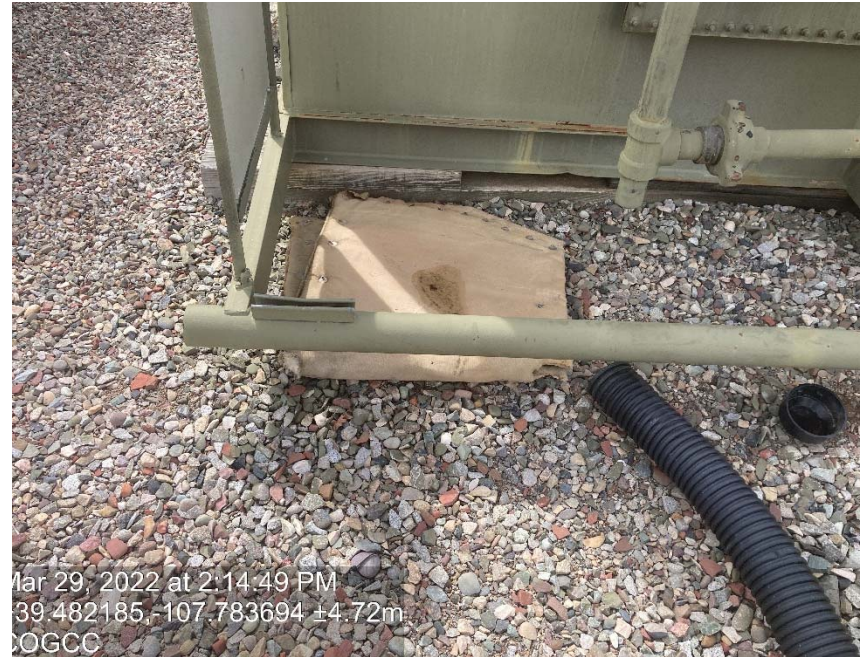
Open ended pipe and debris
