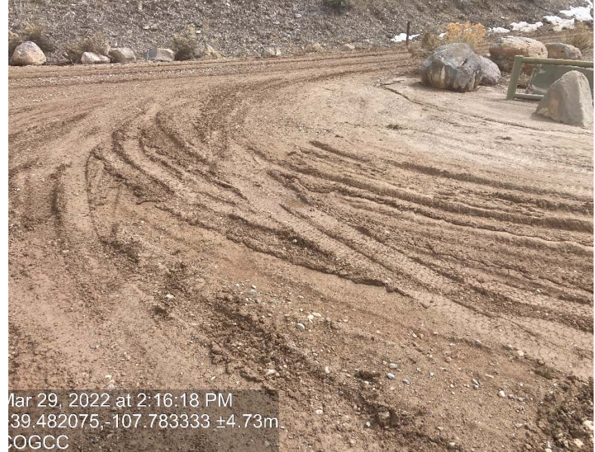
Lack of stabilization/compaction
