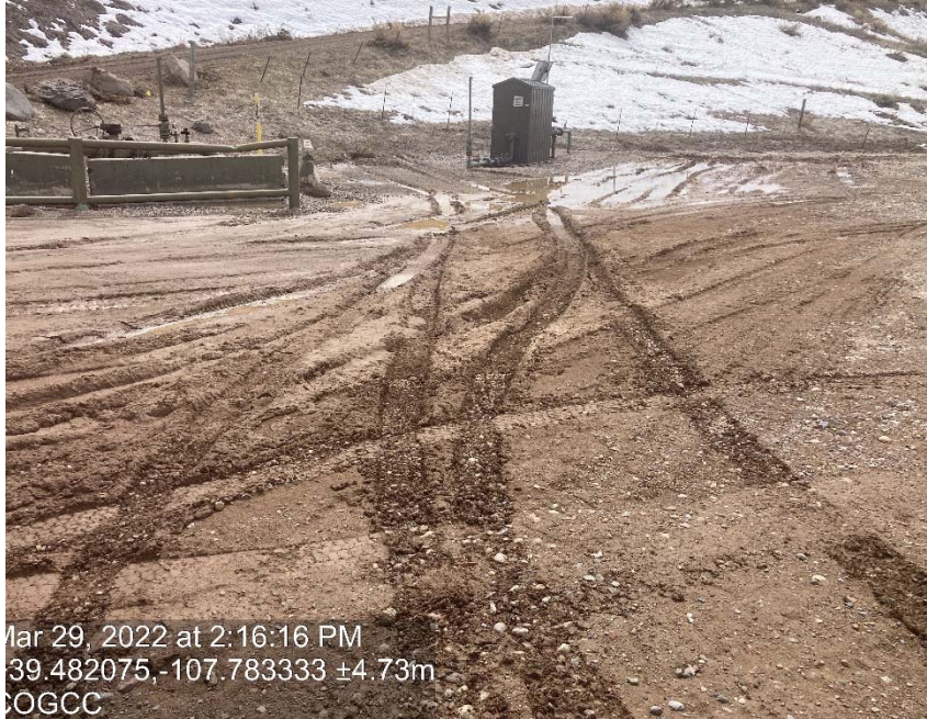
Lack of stabilization/compaction
