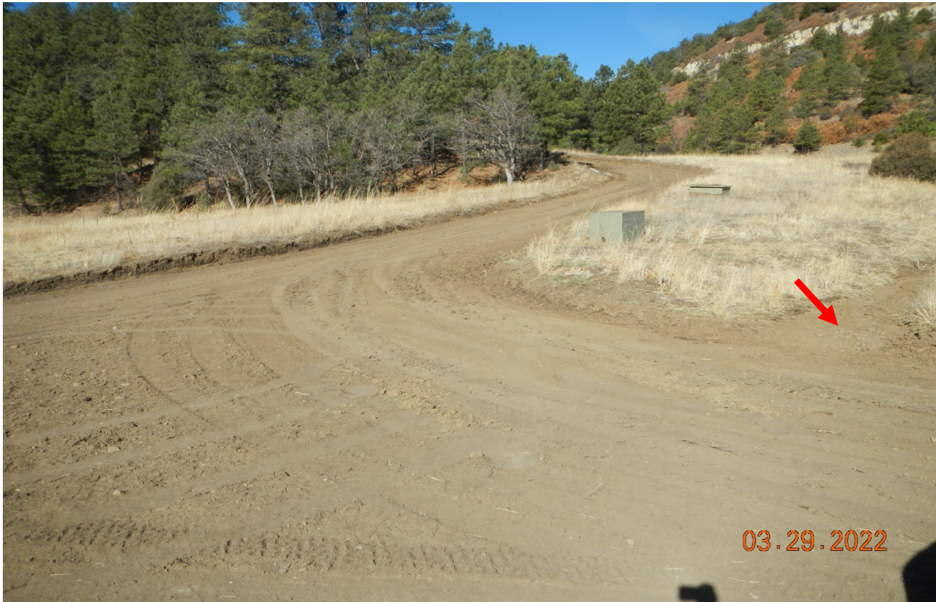
Photo 2. Facing west toward the access road ascending the hillside. The road has been graded. The culvert inlet shown at red arrow and the outlet is shown in photo 4.
