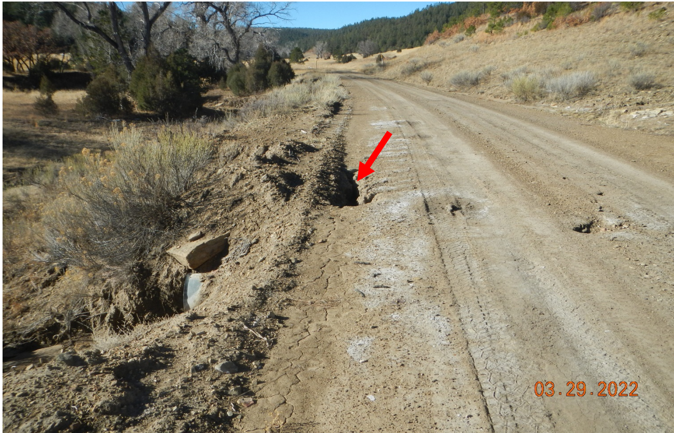
Photo 1. Facing southwest along the main road in the canyon. The road has been graded however, there is still culvert maintenance needed. Red arrow points to erosion undercutting by the culvert which will end up eroding the culvert outlet.
