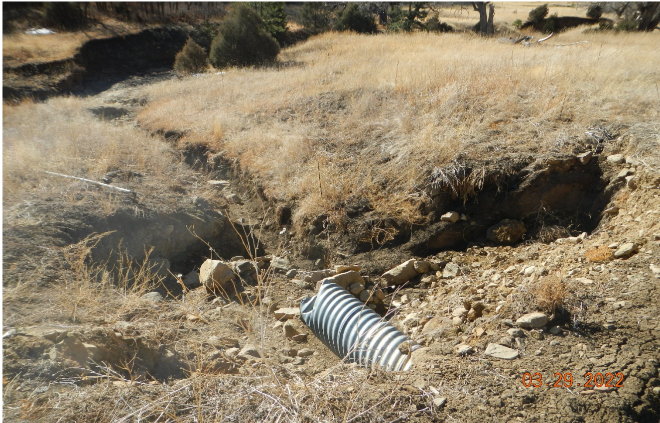
Photo 3. The culvert outlet is eroded and does not have outlet protection. Previous corrective action not completed.
