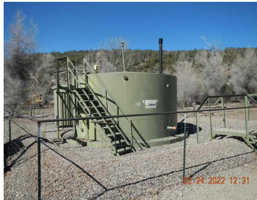
286 bbl. heated steel AST.
