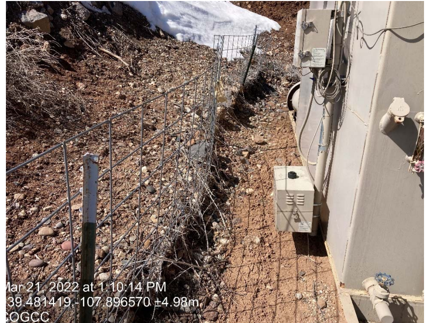
Lack of stabilization/compaction
