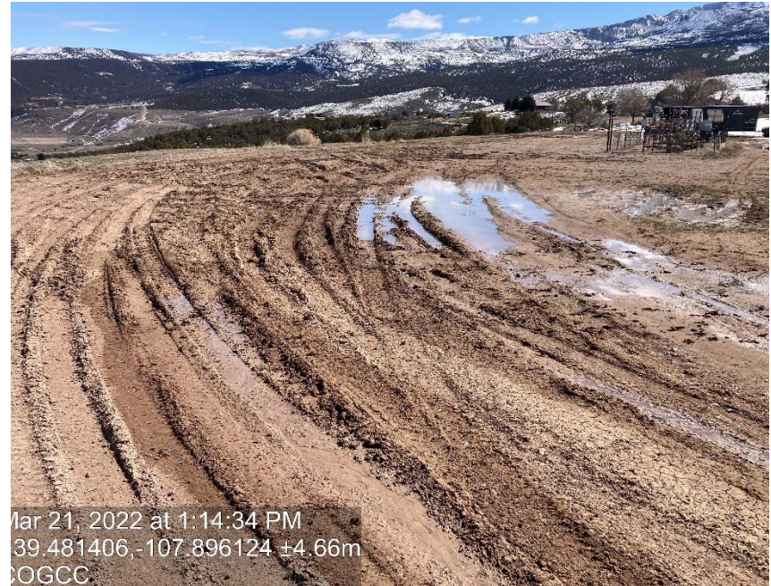
Lack of stabilization/compaction
