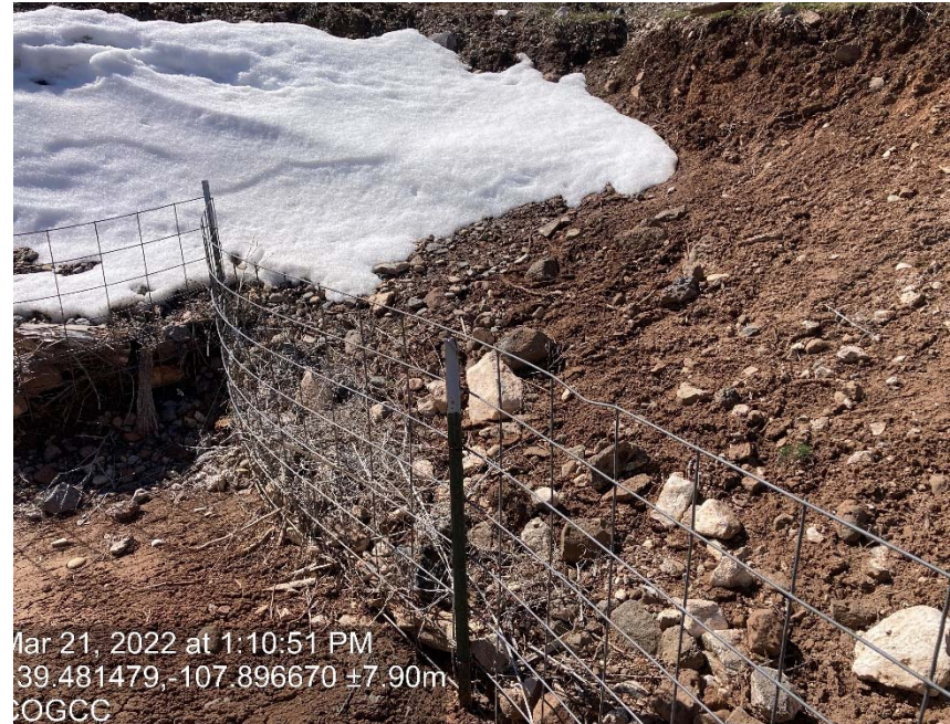
Lack of stabilization/compaction
