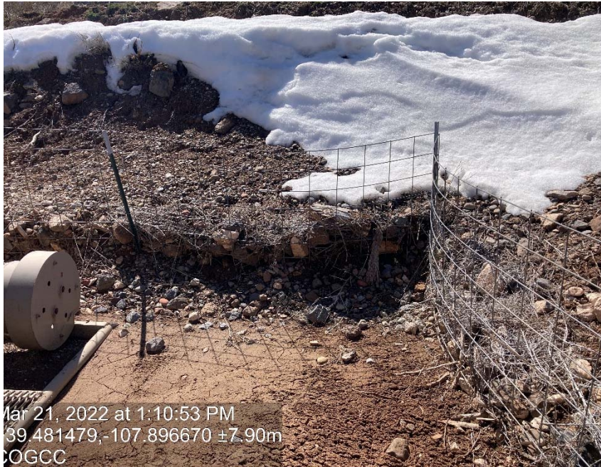
Lack of stabilization/compaction
