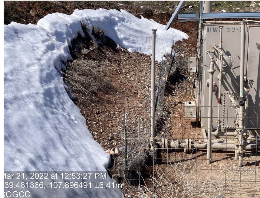
Lack of stabilization/compaction
