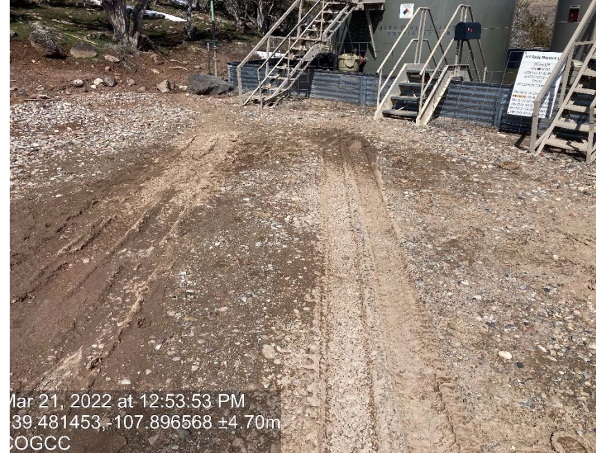
Lack of stabilization/compaction
