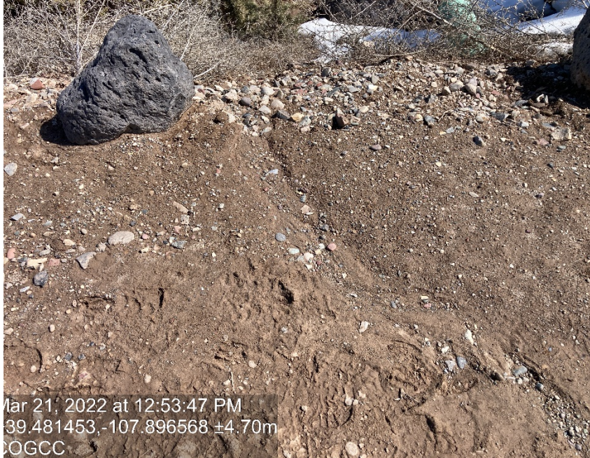
Lack of stabilization/compaction/erosion and sediment migration
