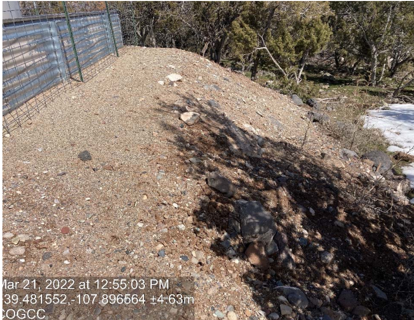
Lack of stabilization/compaction
