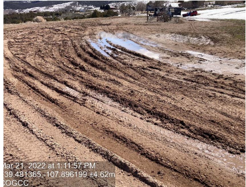
Lack of stabilization/compaction
