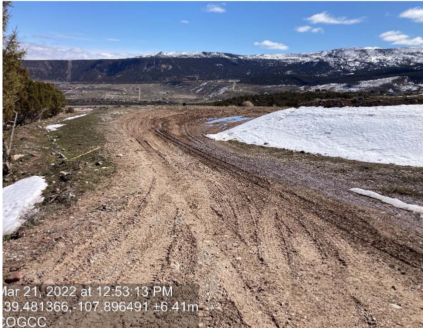
Lack of stabilization/compaction
