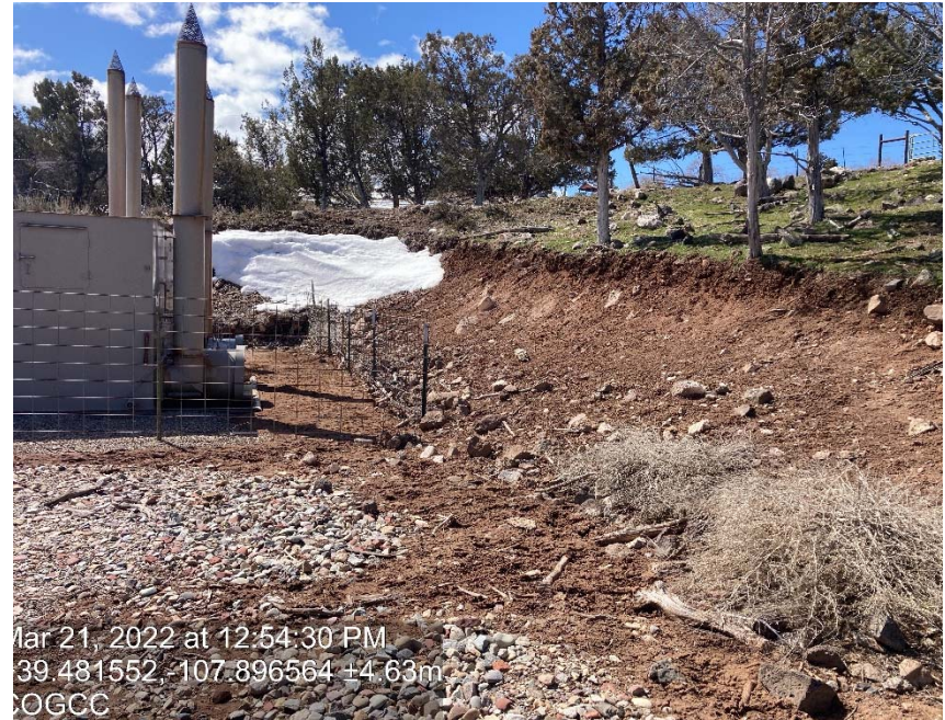
Lack of stabilization/compaction
