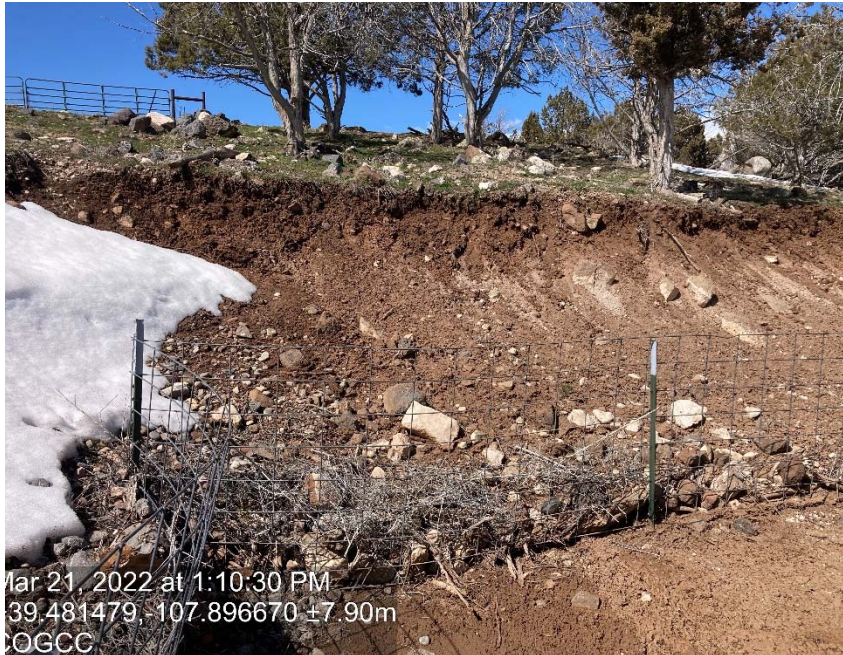
Lack of stabilization/compaction
