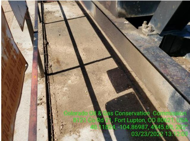
**Photo 7 Stained cement at pump jack base where the seal was leaking.**
