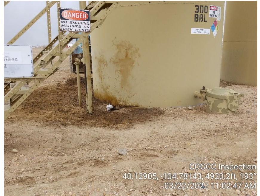
Photo 4 – Spill source on east side of crude tank.
