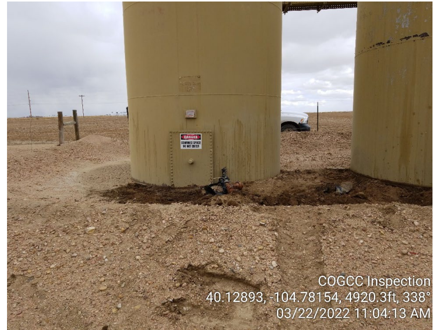
Photo 2 – Spill area on south side of produced water tank.
