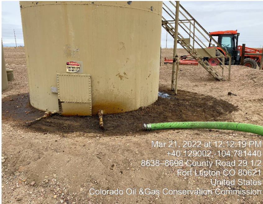
Photo 9 – Active spill observed by COGCC inspector 3/21/2022.
