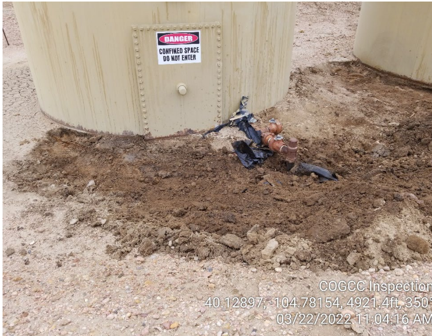
Photo 5 – Spill area on south side of produced water tank.
