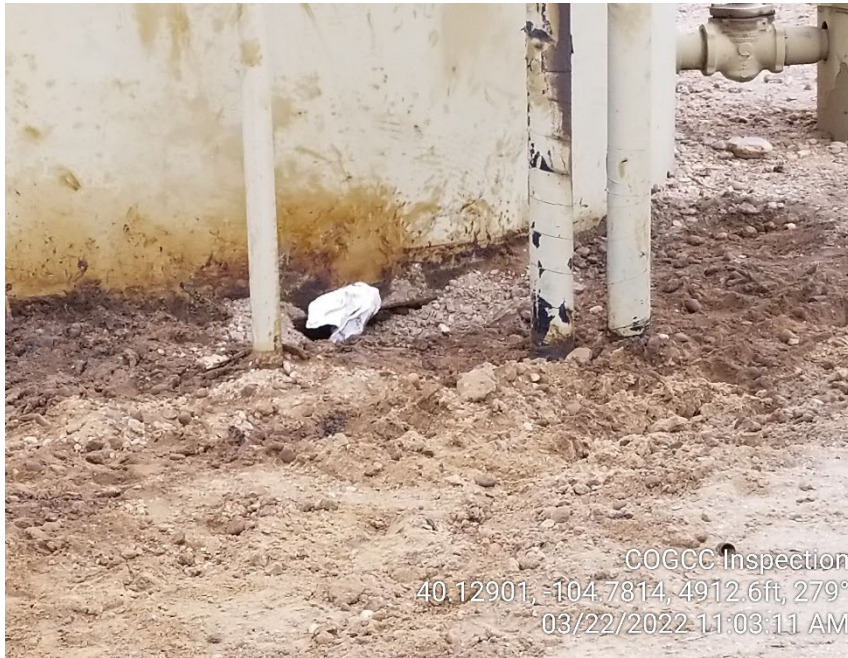
Photo 3 – Spill source on east side of crude tank.
