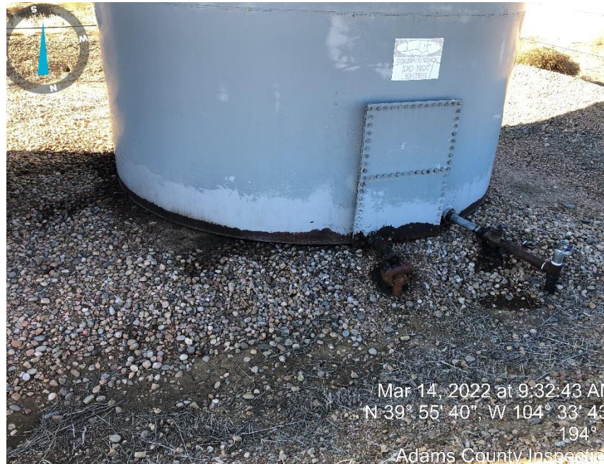
Photo #5 Stained soil around the west crude tank, stains are on the north side.
