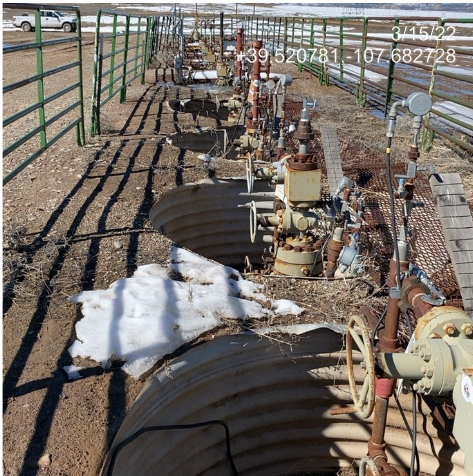
Photo 4. Photo taken from the well equipment facing west shows BMPs to prevent wildlife access to the well cellars were missing or insufficient.
