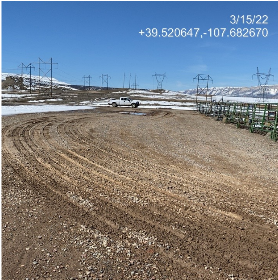
Photo 7. Photo taken from the east of the Location facing west shows rutting occurring on the pad.
