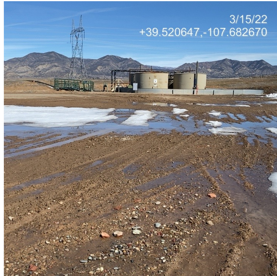
Photo 8. Photo taken from the east of the Location facing north shows rutting occurring on the pad.
