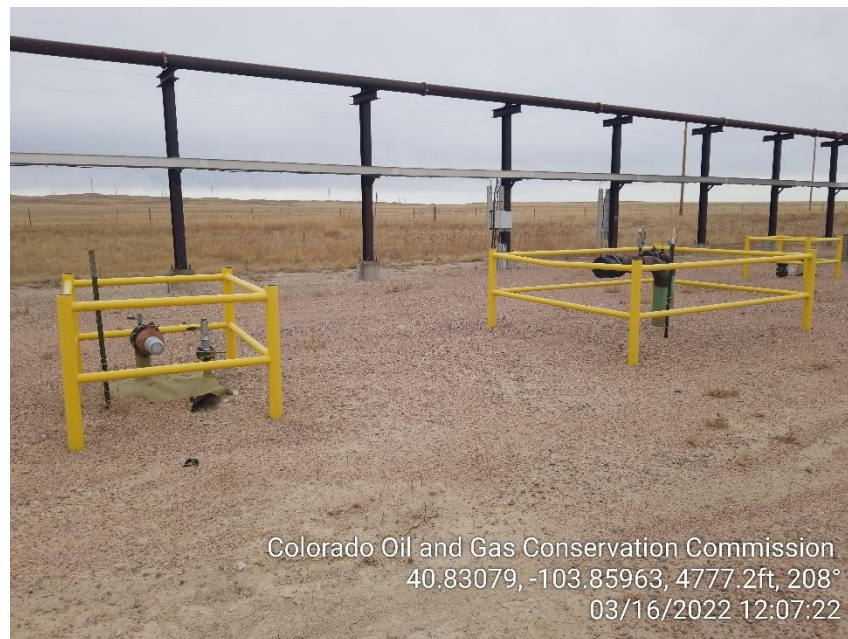
Photo 22 – Unmarked Risers on North Side
