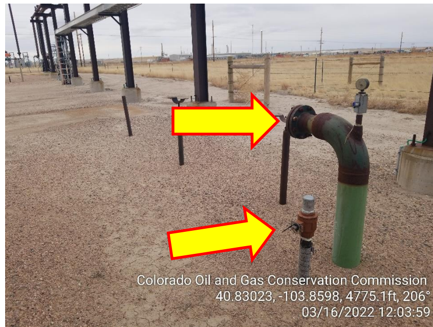
Photo 14 – Unmarked Risers on West side of Location
