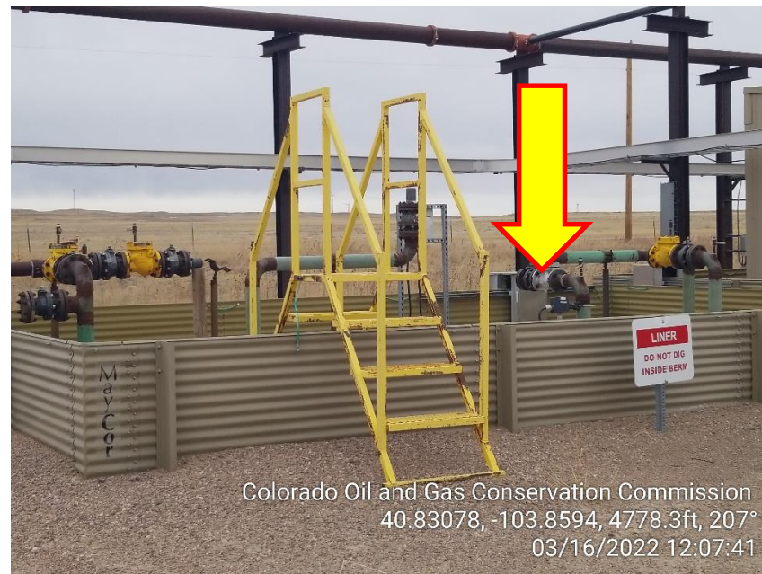
Photo 24 – Unmarked Risers on North Side
