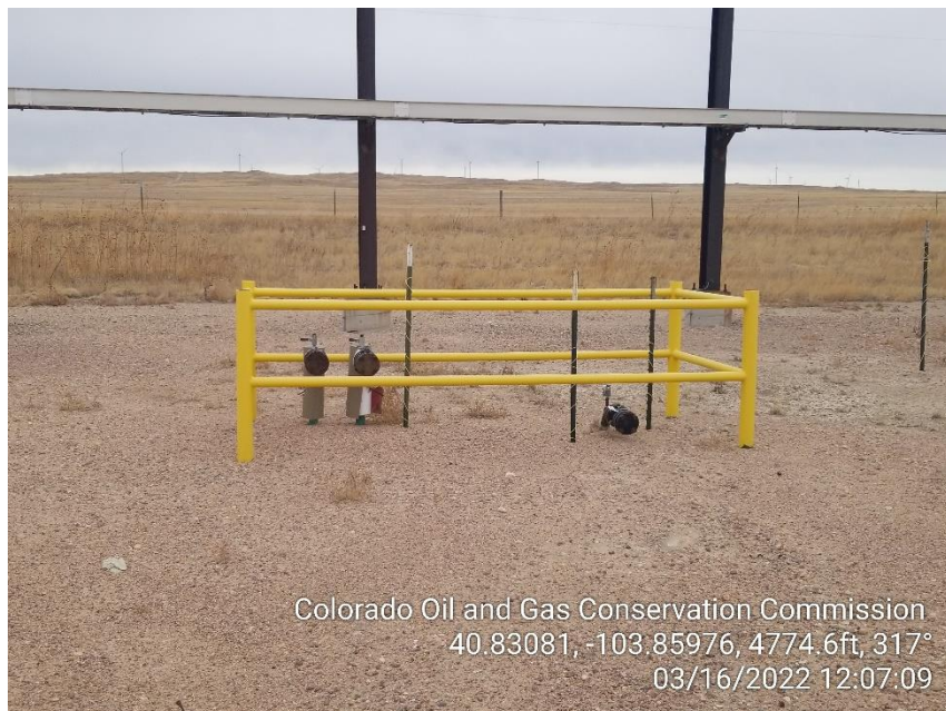
Photo 21 – Unmarked Risers on North Side
