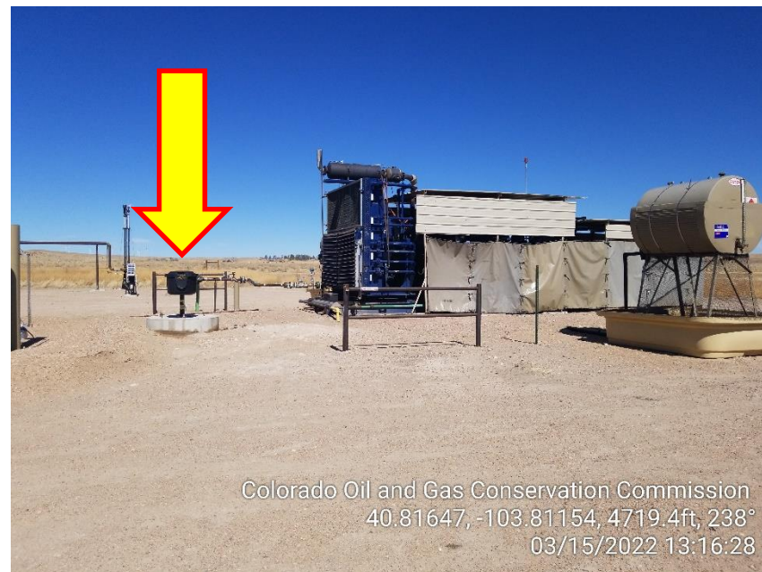
Photo 6 – Compressor – Drain Pit missing Labels
