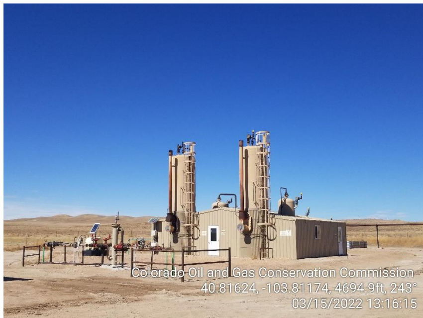
Photo 5 – Heater Treaters
