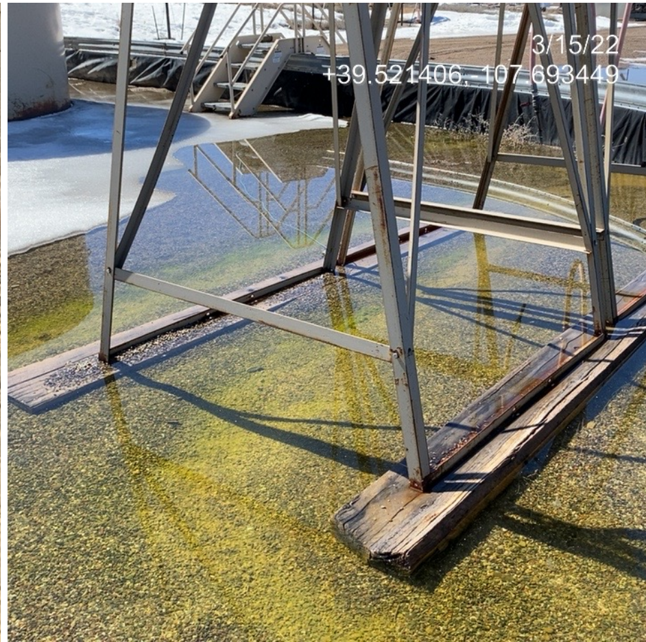
Photo 3. Photo taken from the north of the tank battery shows potentially impacted fluids throughout the secondary containment area of the tank battery.
