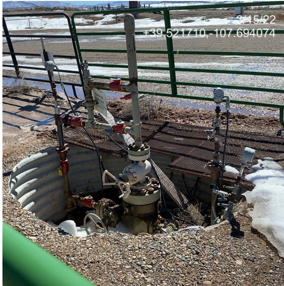
Photo 4. Photo taken from the well area shows BMPs to prevent wildlife access to the well cellars were missing or insufficient.
