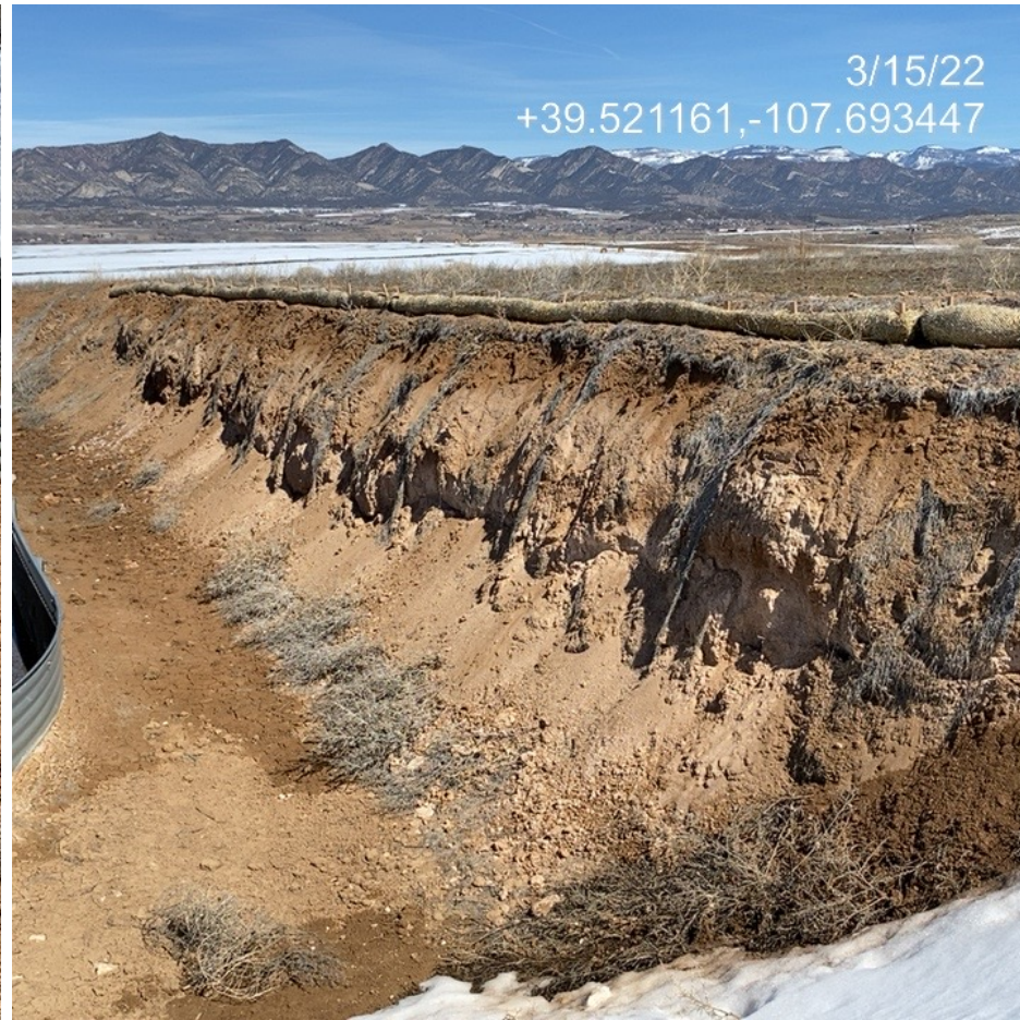
Photo 6. Photo taken from the southeast of the Location shows unstable soils of the cut slope.
