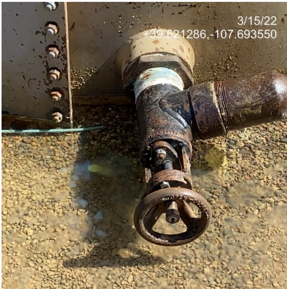
Photo 2. Photo taken from the northwest of the tank battery shows an unknown substance below the tank valve.
