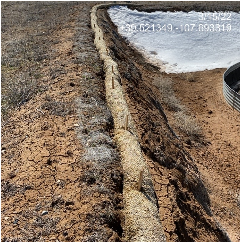
Photo 5. Photo taken from the east of the Location at the top of the cut slope shows a straw wattle has been installed to prevent run on.
