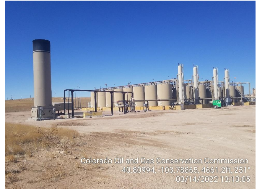
Photo 2 – Tank Battery
