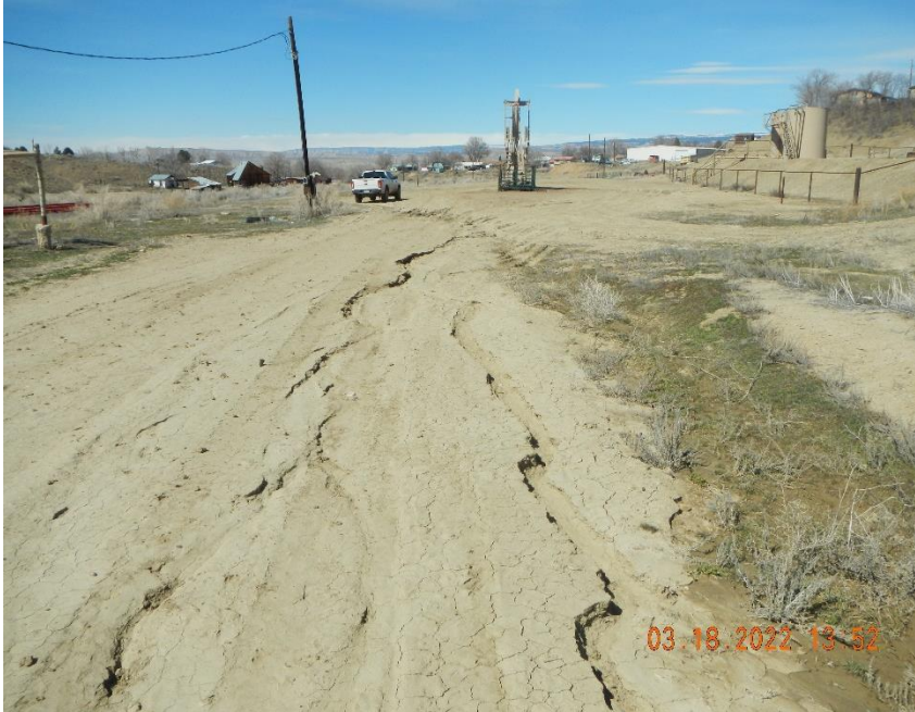
Storm water damage of access road and moving across south end of location.
