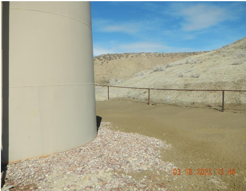
Sediment coming off hillside behind tank battery berm and collecting sediment and stormwater in berm.
