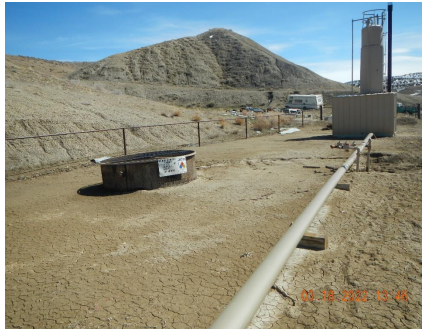
Subsidence of tank ground base. Base of berm is marshy.
