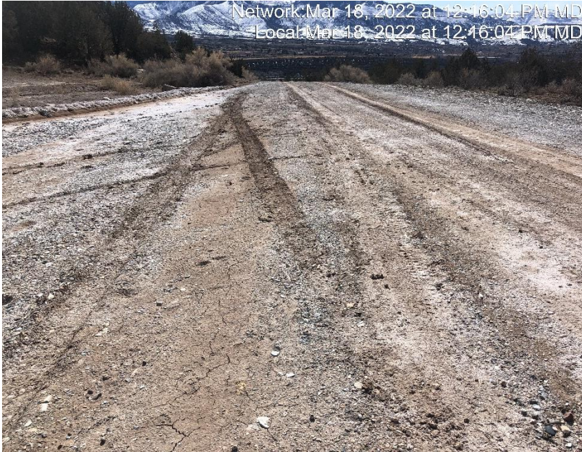
Photo #6247 Insufficient tracking BMP at entrance to location.
