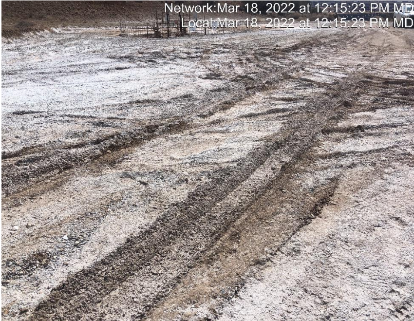
Photo #6245 Location lacks stabilization.
